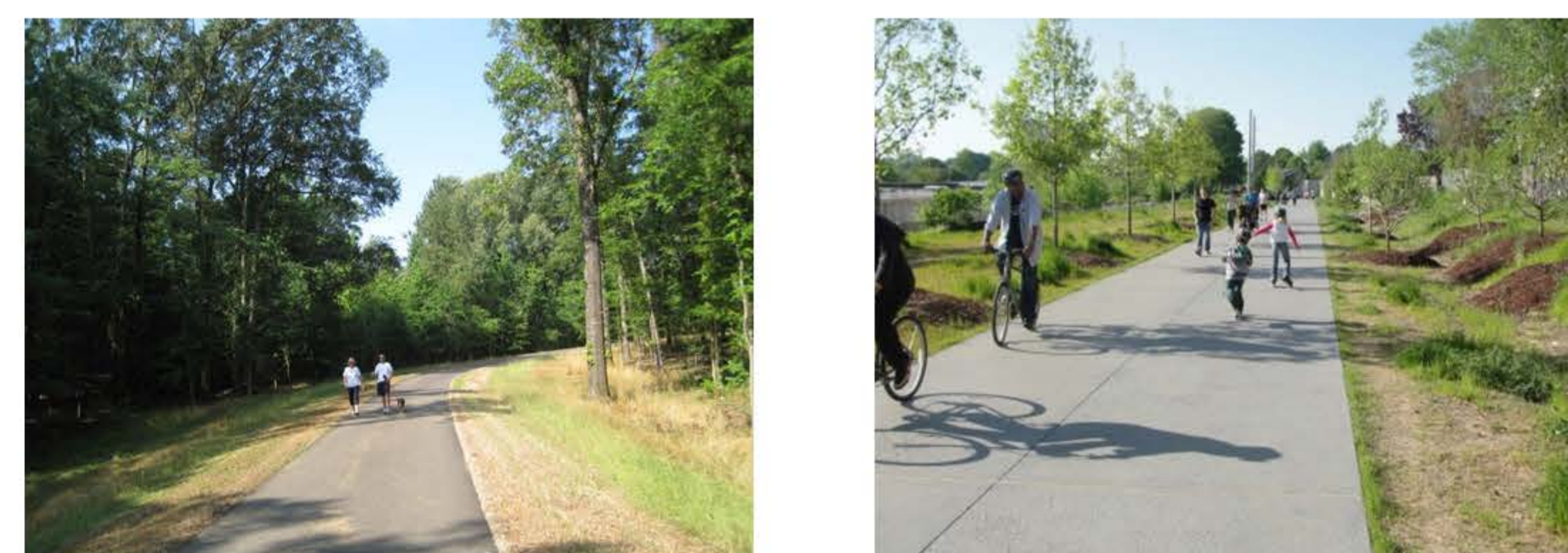
The images above provide an example of an approximately 10 foot wide paved path with both bicycles and pedestrian use
