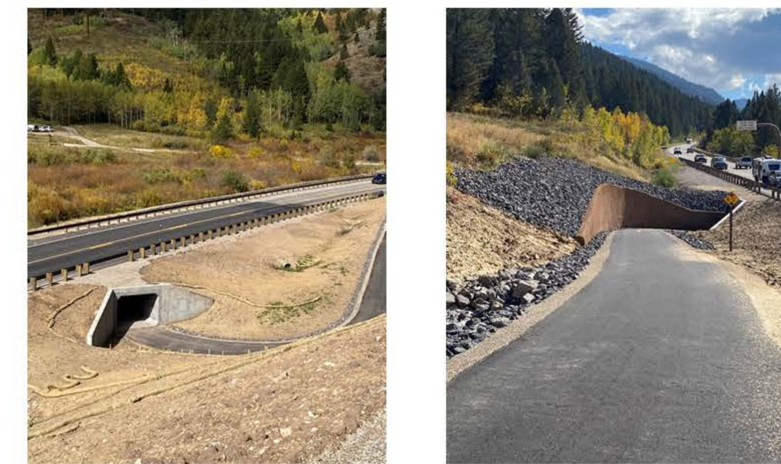
Centennial Trail Grade Separated Crossing (Pedestrian Tunnel) at Idaho-Wyoming Border (ID-33 and WY-22)
