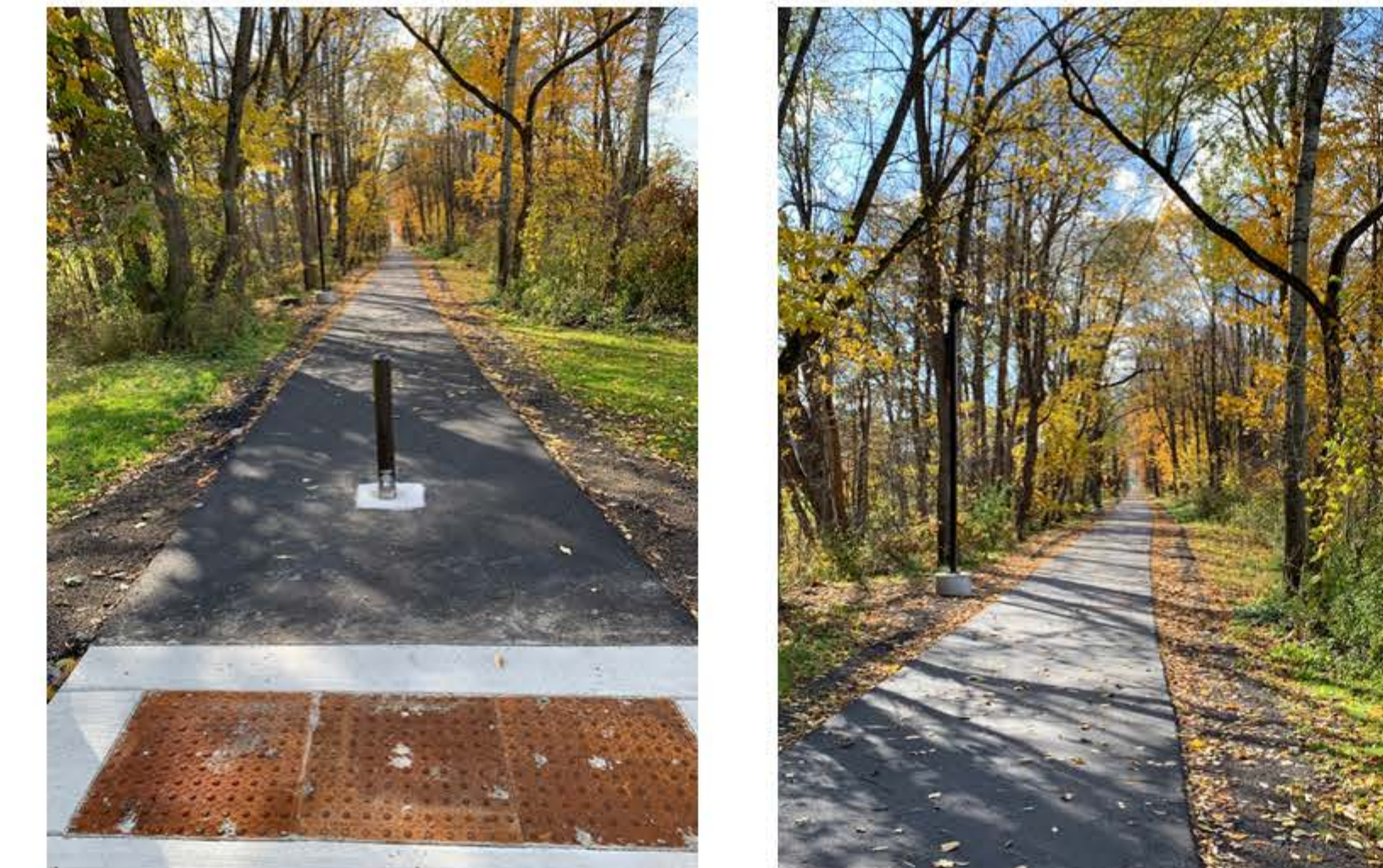
The images above provide an example of an approximately 10 foot wide paved path, including features for the end of a trail segment (top left)
