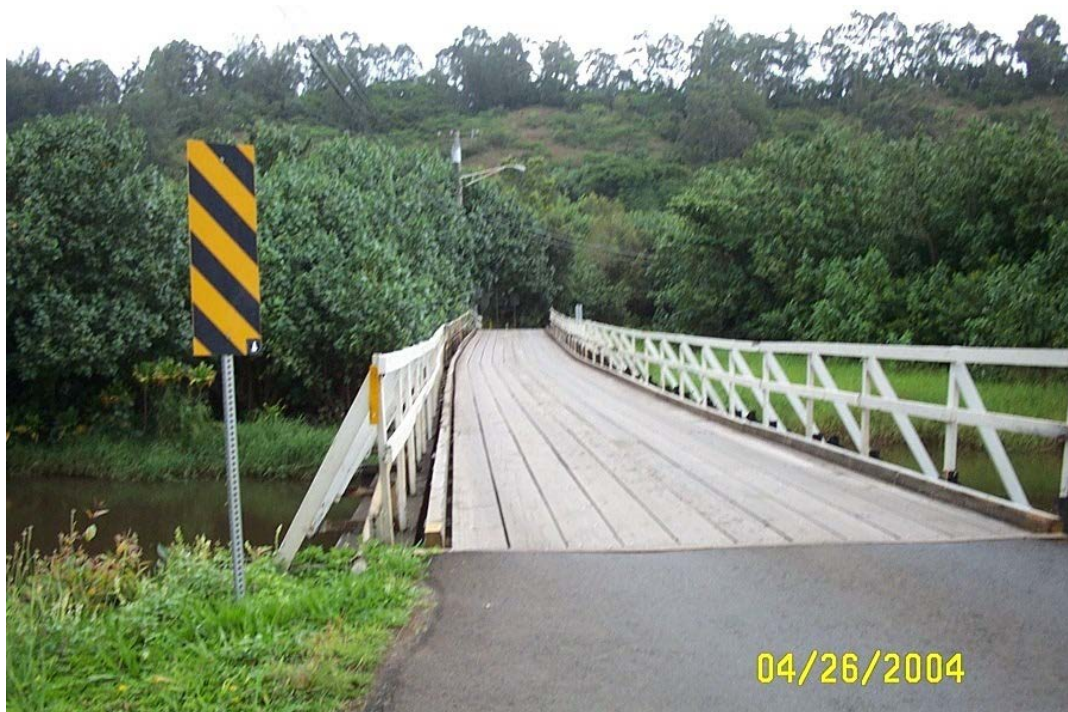
1957 Bridge 3 – Approximately 146-feet in length and 11-feet in width.
