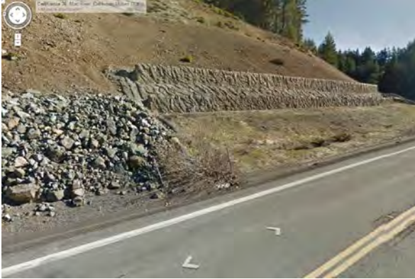
Rock buttress and rock-faced retaining wall east of project area.
