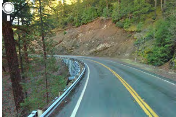
Guardrail, typical cut slope, and crib wall (metal retaining wall) east of project area.
