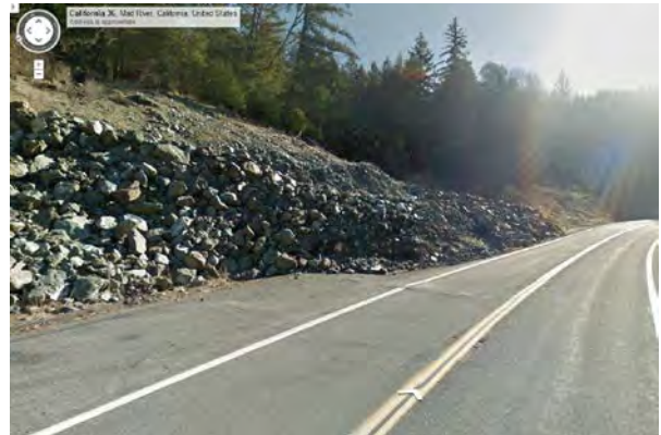
Rock buttress slide into SR 36 shoulder, east of project area.
