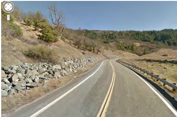
Guardrail and sustained buttress along SR 36 ascent east of project area.
