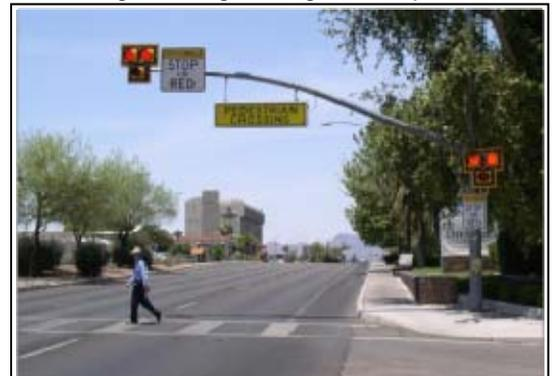
The alternating flashing red phase allows the delay to traffic to match the actual crossing needs of the pedestrians. Drivers can proceed with a stop-and-go operation during the flashing red phase. If pedestrians need more time, then the drivers remain stopped until they finish crossing. The ability to balance the pedestrian needs with driver delay is a valuable component of the HAWK treatment.
