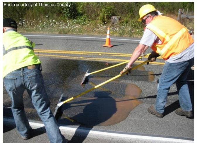
*Thurston County’s crew prepared the resin, applied it to the road, and covered it with a specialized calcined bauxite aggregate at this HFST project in 2014.*
