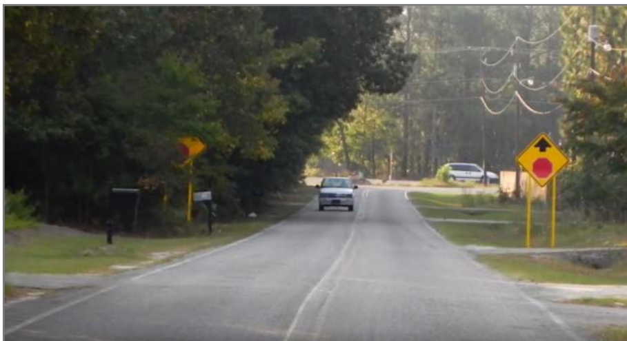
Enhanced signage is one systemic approach to improve safety on rural roadways. (Source: FHWA)
