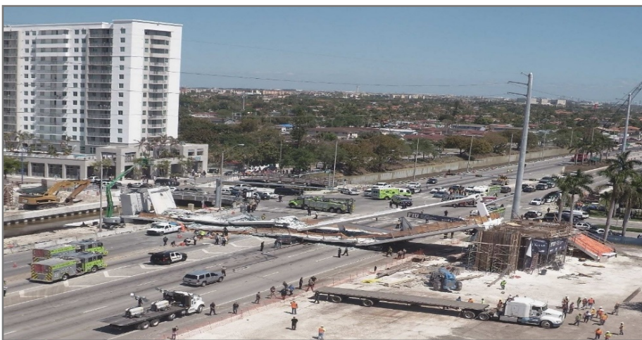
Bridge collapse. (Source: NTSB)
