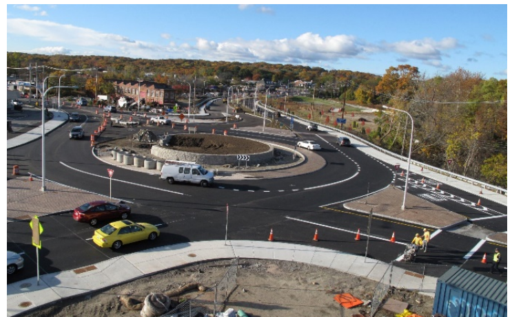
Aerial view of the new Apponaug Village roundabout during final construction. Source: RIDOT
