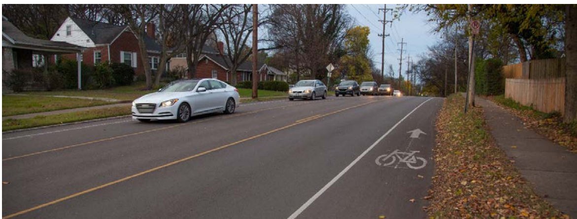
A Road Diet with bicycle accommodations. (Source: FHWA)
