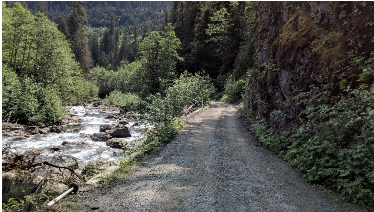
Figure 15: Narrow Width of Existing Gravel Section
