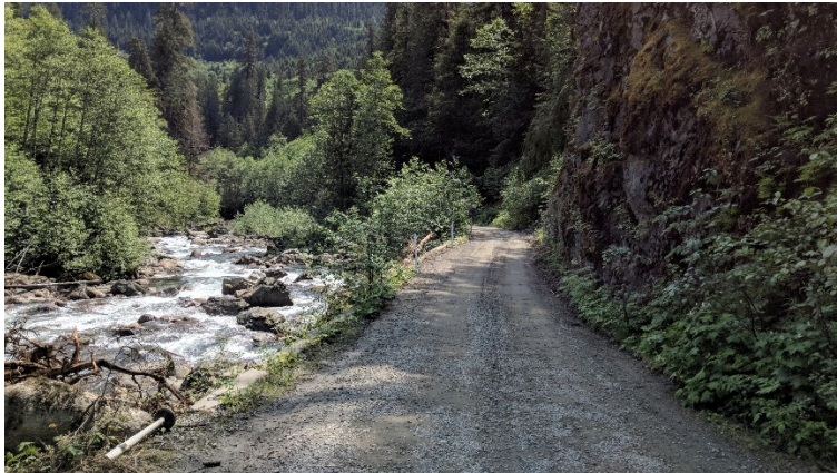
Figure 15: Narrow Width of Existing Gravel Section
