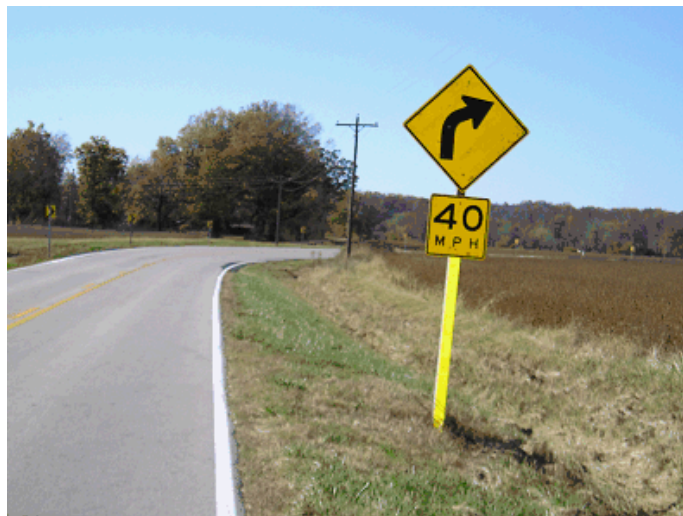
Photo 1. 4-inch edge-line markings were added to this horizontal curve along a rural Missouri highway. Source: Missouri DOT.
