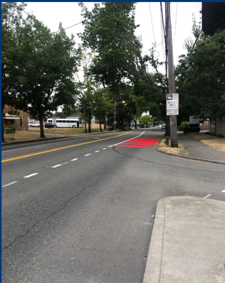
Figure 1. Photograph. Newly installed bus lane on Rainier Avenue South at South Cloverdale Street.
