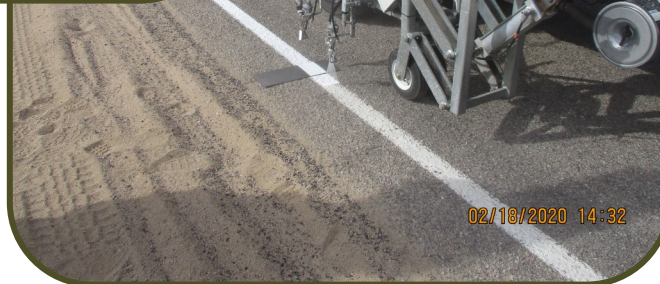
Testing the paint thickness.
