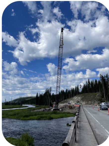
Crane and sheet pile driving.
