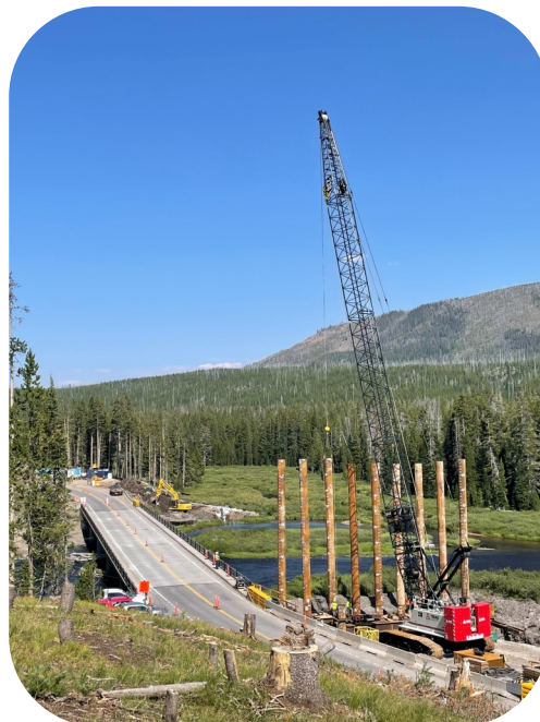
View of the project.
