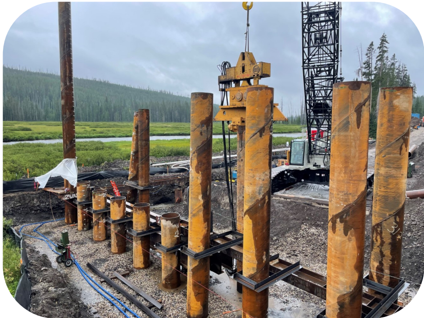
Pipe pile driving on the south side.
