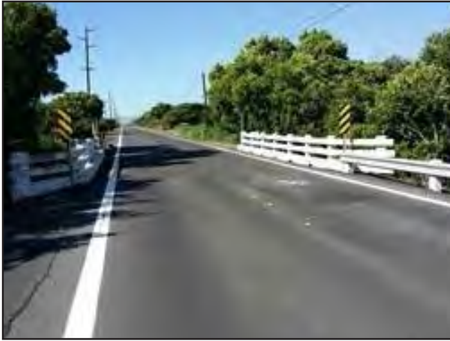
Photo 1. Hilea Bridge asphalt deck, view to southwest
