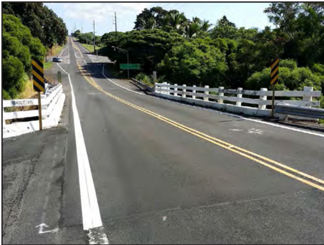
Photo 1. Ninole Bridge, view to northeast
