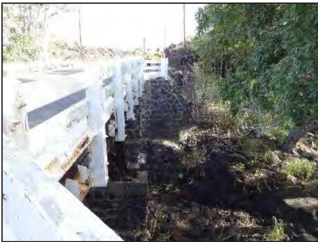
Photo 3. Hilea Bridge, view to northeast
