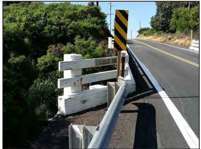
Photo 2. Ninole Bridge, view to southwest
