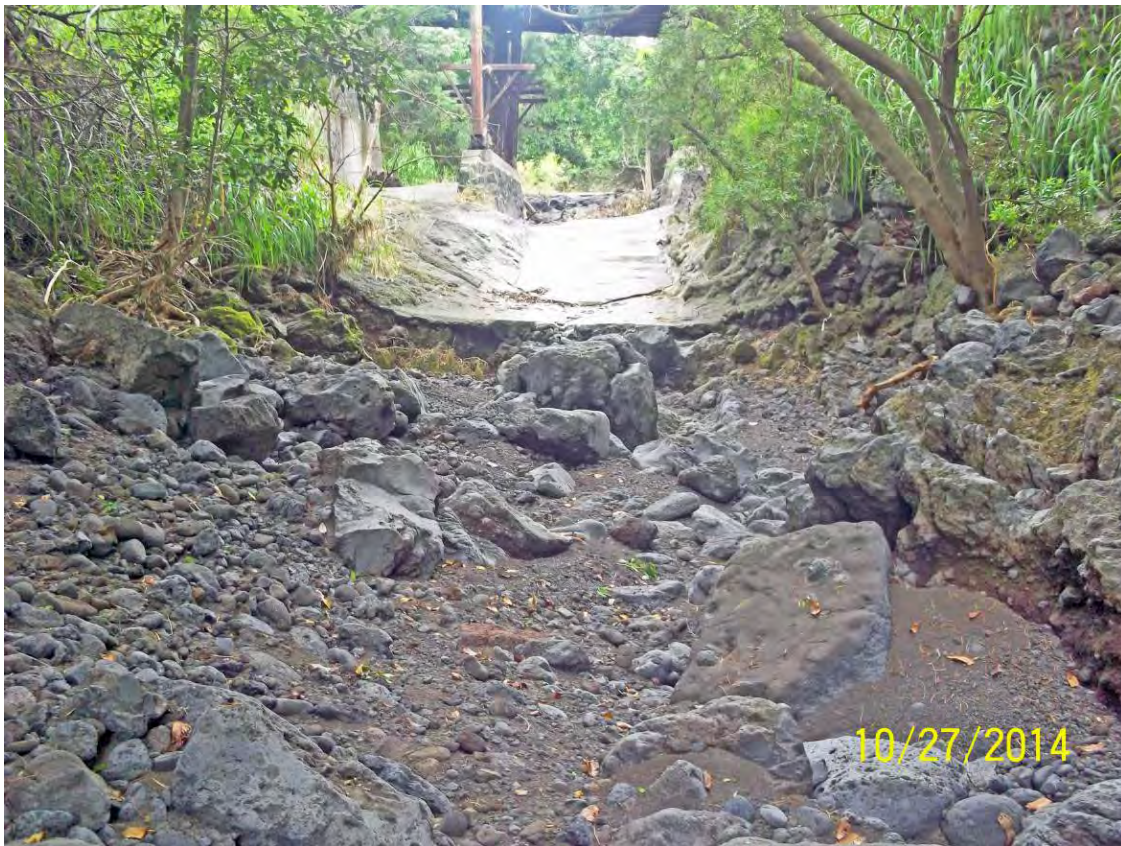
Figure 9. Sand and gravel deposition is apparent in the gulch downstream of the spillway under the middle bay of the bridge on Nīnole Gulch.
