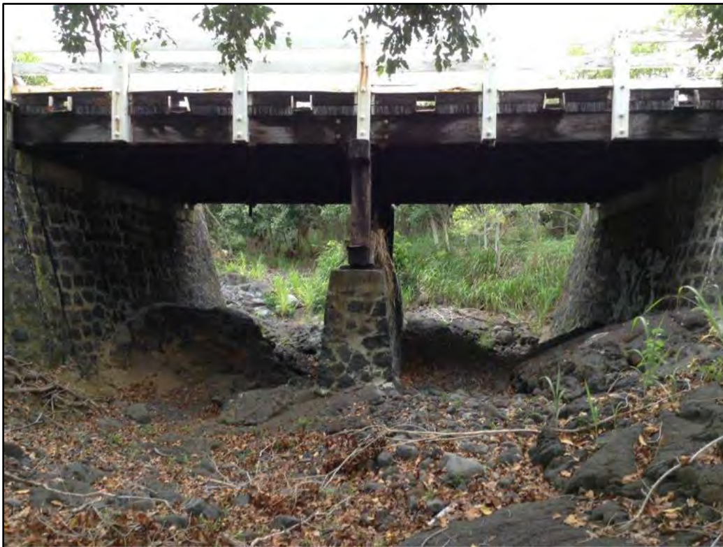
Figure 37. Hīlea Bridge (SIHP # 50-10-74-30298) timber columns and footings, view to west
