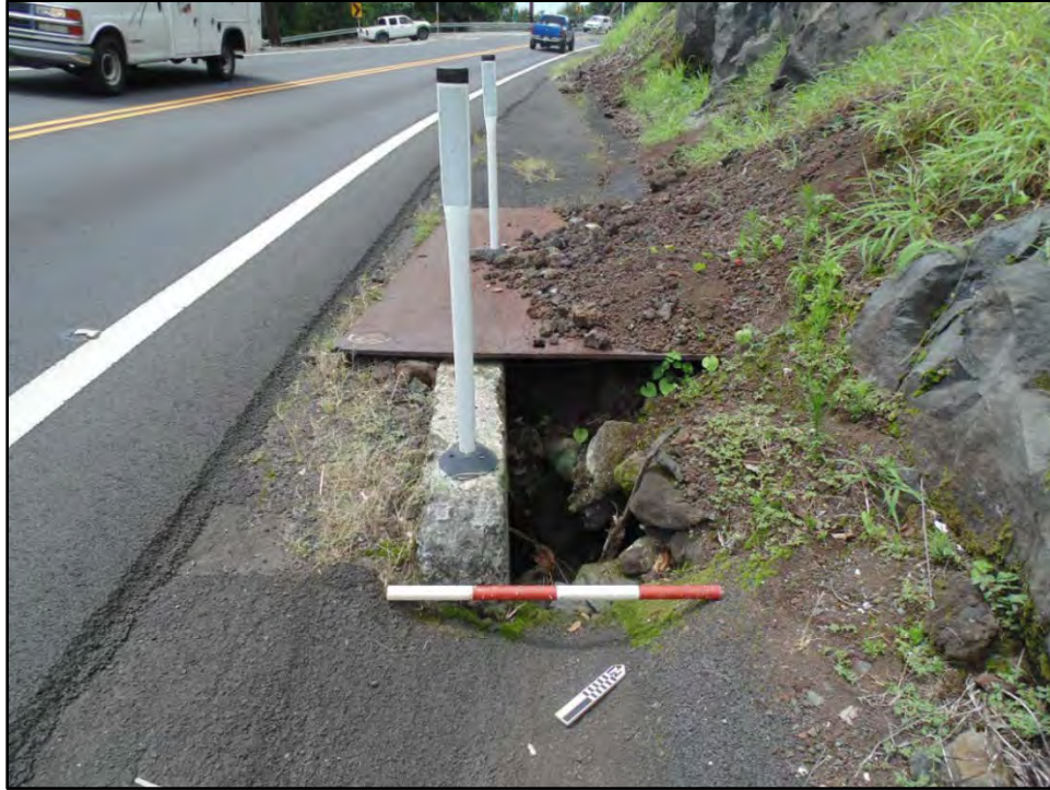
Figure 27. SIHP # 50-10-47-30187 Feature E concrete culvert inlet in South Kona, view to northeast (Clark et al. 2014:59)
