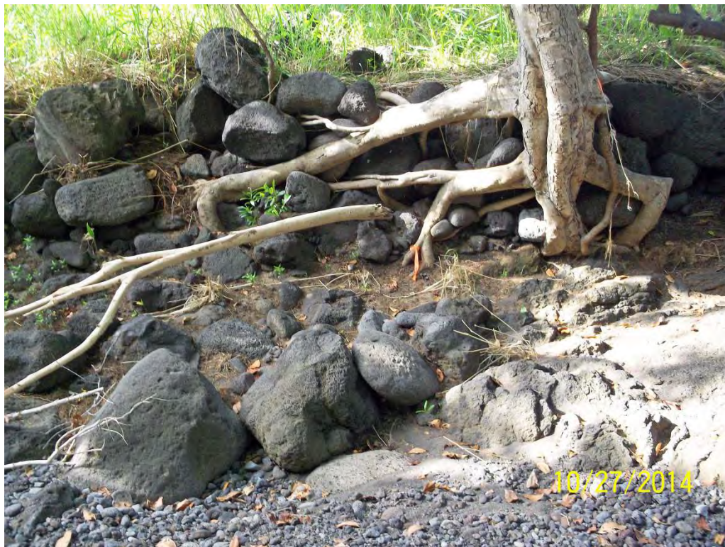
Figure 7. The right side of Hīlea Gulch has been built up in a berm to protect the former sugar cane fields from freshets.
