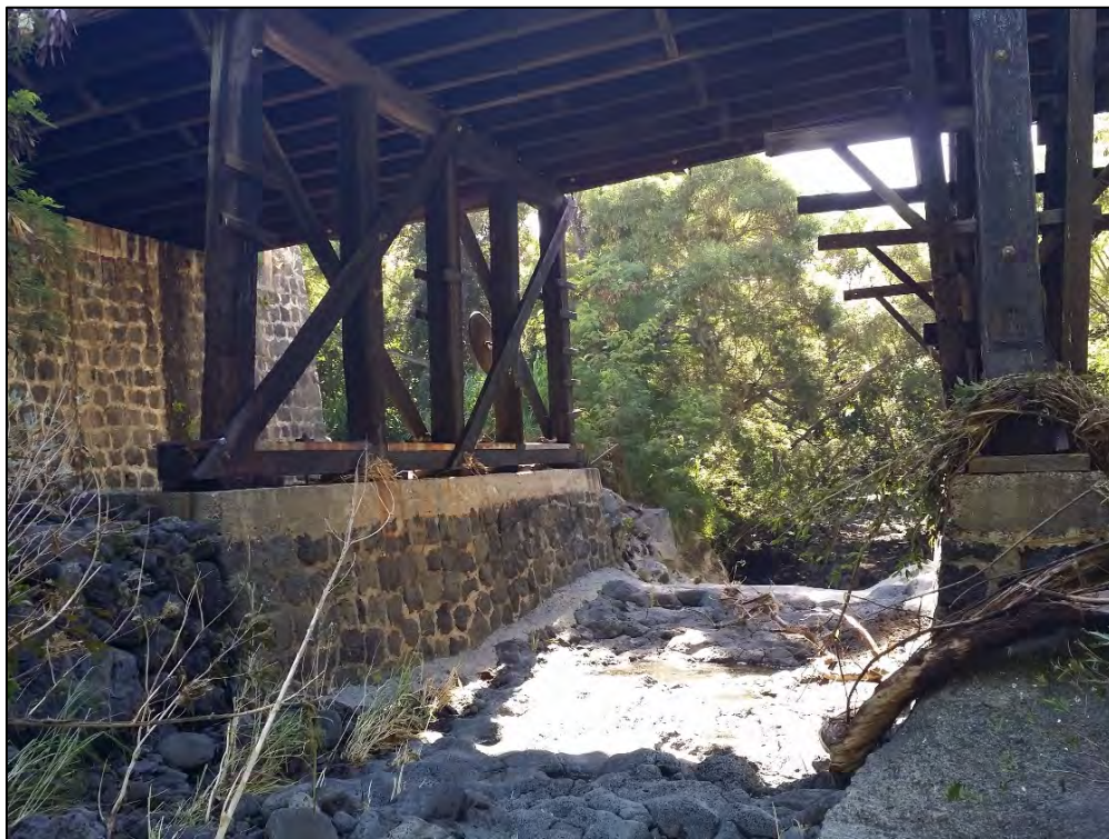
Figure 35. SIHP # 50-10-68-30299, Nīnole Bridge timber columns and footings, view to northwest
