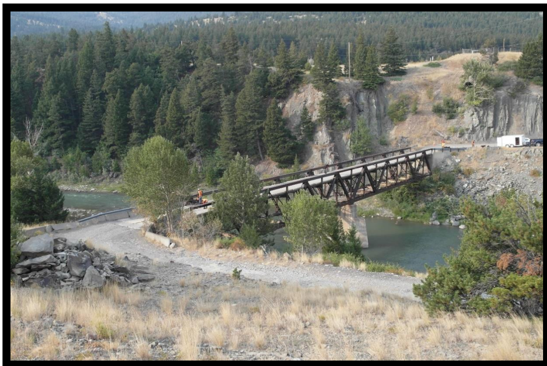
Photo 2 – The Sun River Bridge looking downstream. Note the sharp, abrupt angled bridge approaches that limit bridge use and restricts access to Federal lands.
