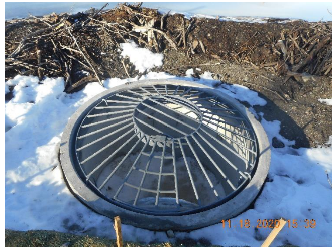
Completed Manhole and Debris Cage at Beaver Pond
