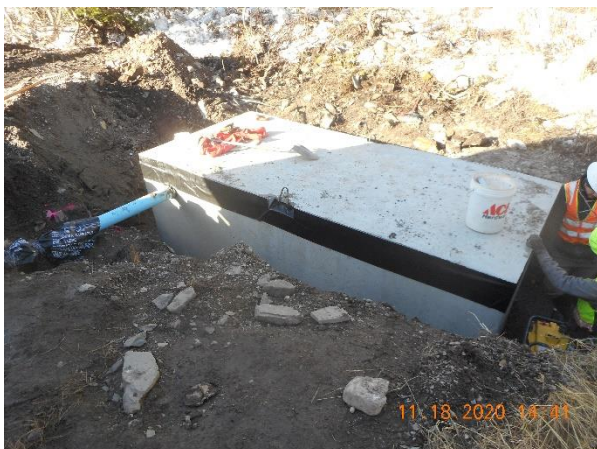
1000 Gallon Tank Installation for Sewer Work
