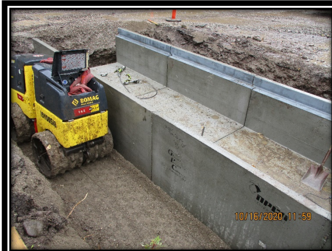
RCB Trench Drain
