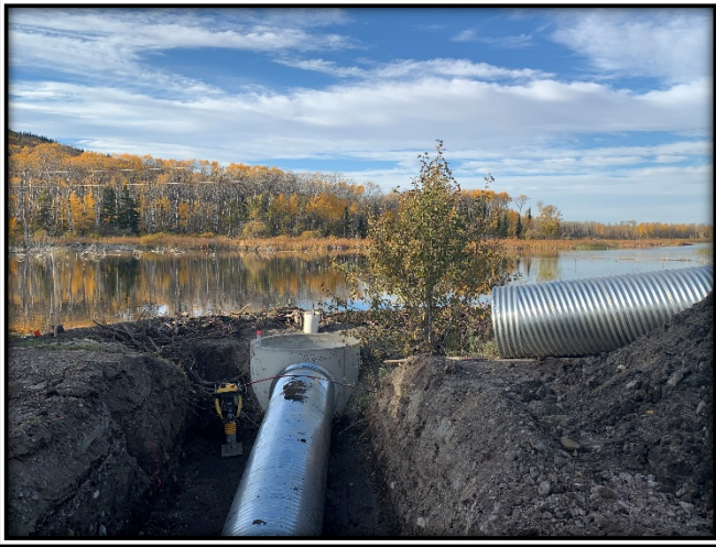
Installation of Manhole and Culvert at Beaver Pond
