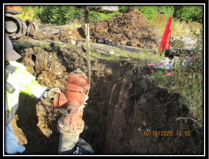
MGH Parking Lot Fire Hydrant Relocation
