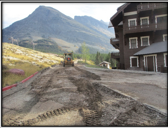
Grading at Many Glacier Hotel Loop Road
