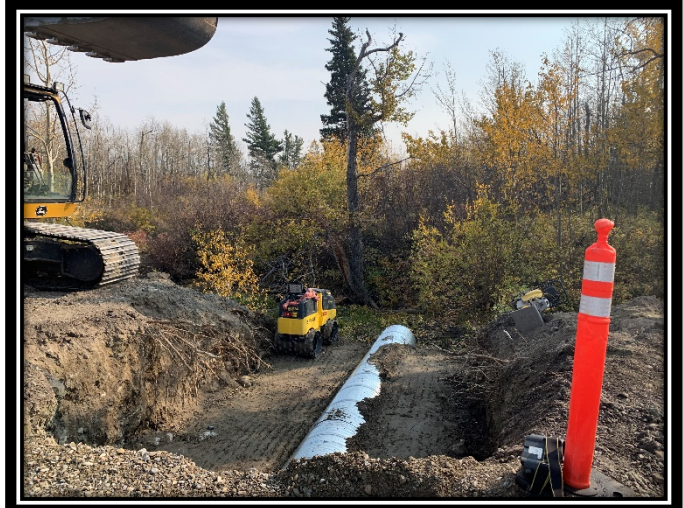
Installation of Culvert on Option X
