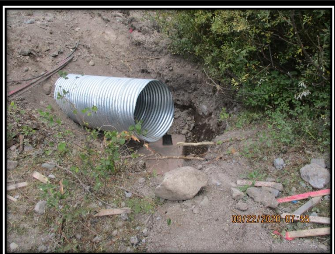
Installation of Culvert at Option X
