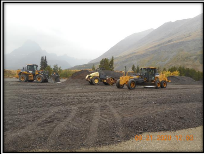
MGH Parking Lot Recycled Aggregate Base
