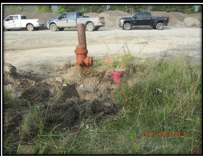
Relocate Fire Hydrant at MGH Parking Lot
