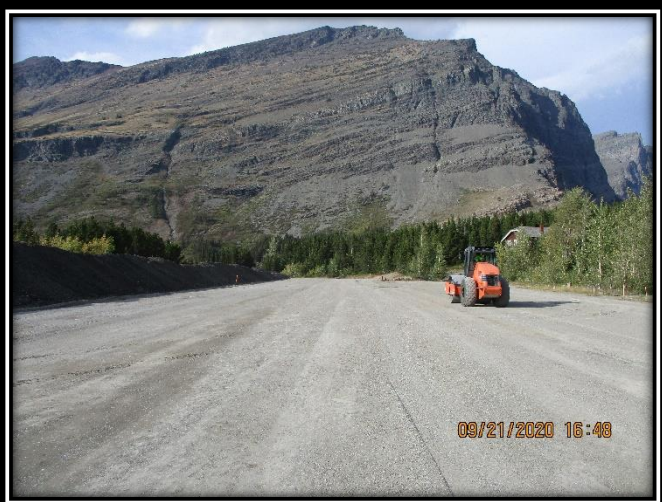
MGH Parking Lot Aggregate Base D Grading
