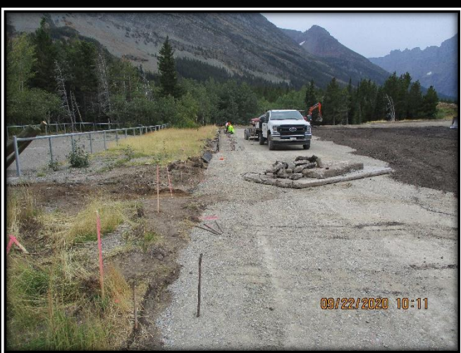
Install Curb and Gutter forms and Recycle Aggregate Base at MGH Parking Lot
