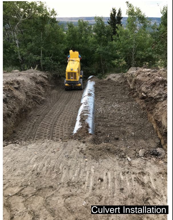
Repair Drainage Structure
