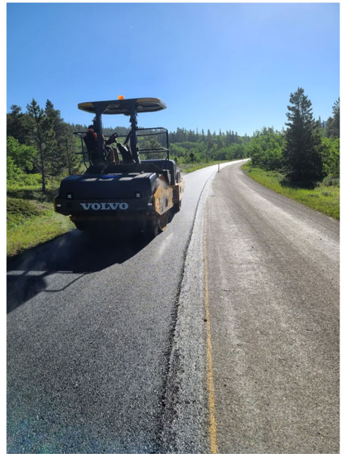
Rollers Compacting Asphalt Mat
