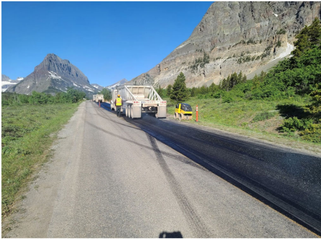
Rollers Compacting Asphalt Mat
