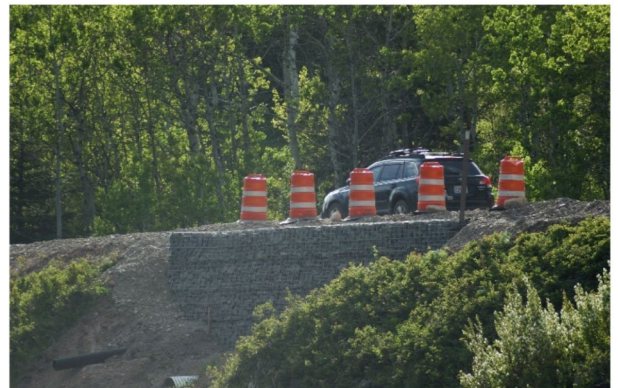
The MSE Retaining Wall on Option X is Complete
