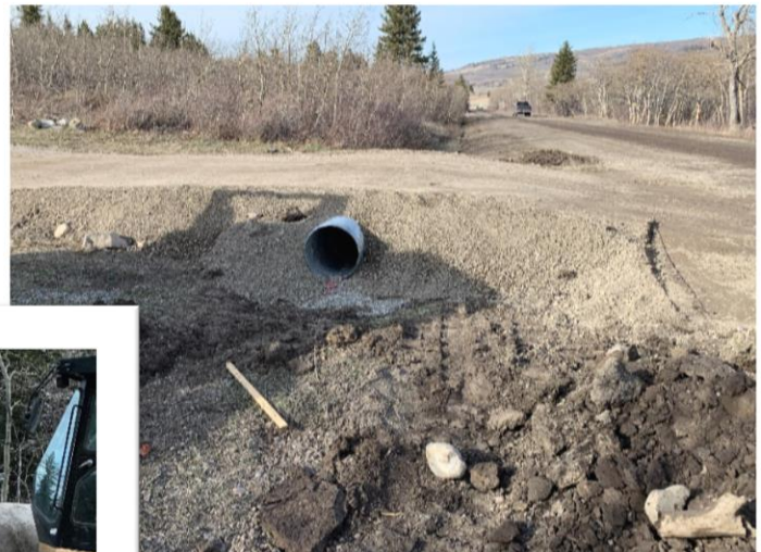
Culverts are Installed at Residential Approaches
