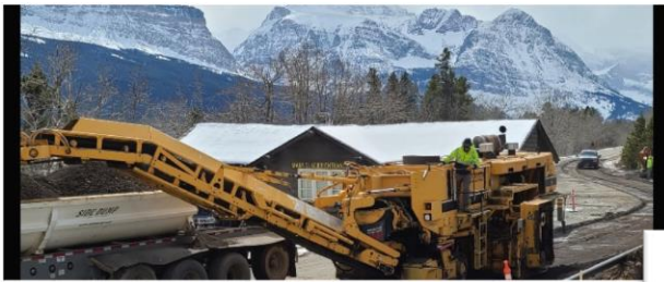
Asphalt is Milled at the Entrance Station
