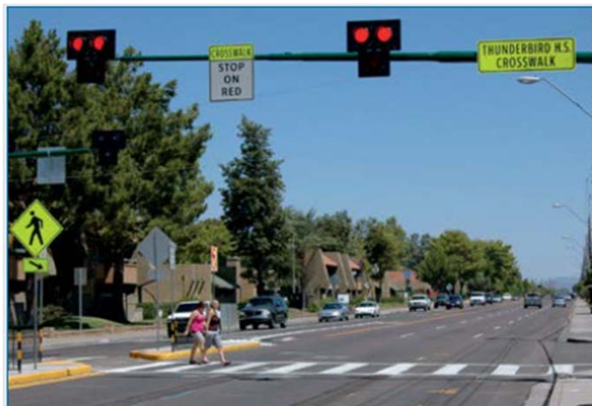
Illustration of a pedestrian hybrid beacon at a mid-block crossing.
