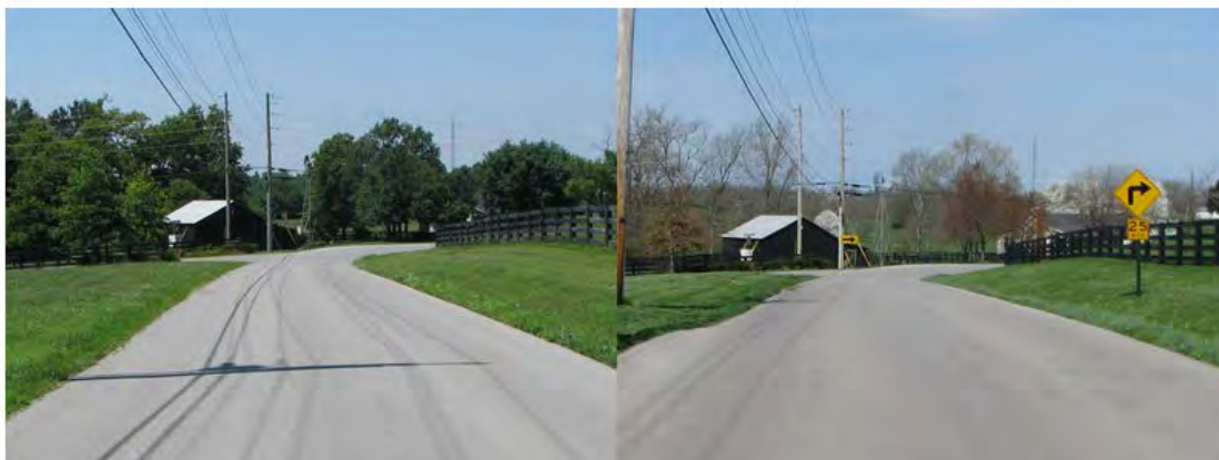
Before and After Curve Warning Countermeasure Installation on Vince Rd.
