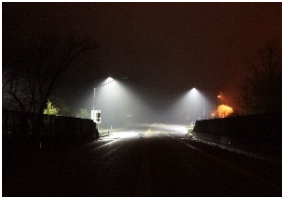
Intersection lighting. (Source: FHWA)
