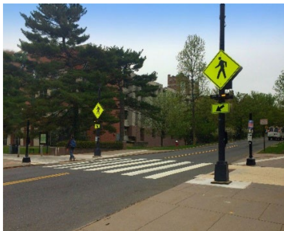
High-visibility crosswalk. (Source: FHWA)
