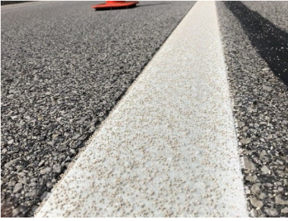
Recessed highly reflective polyurea pavement markings. (Source: PTC)
