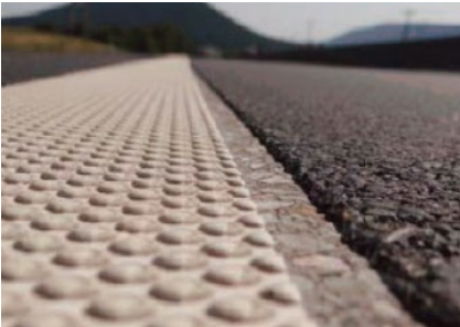
Recessed all-weather tape. (Source: PTC)
