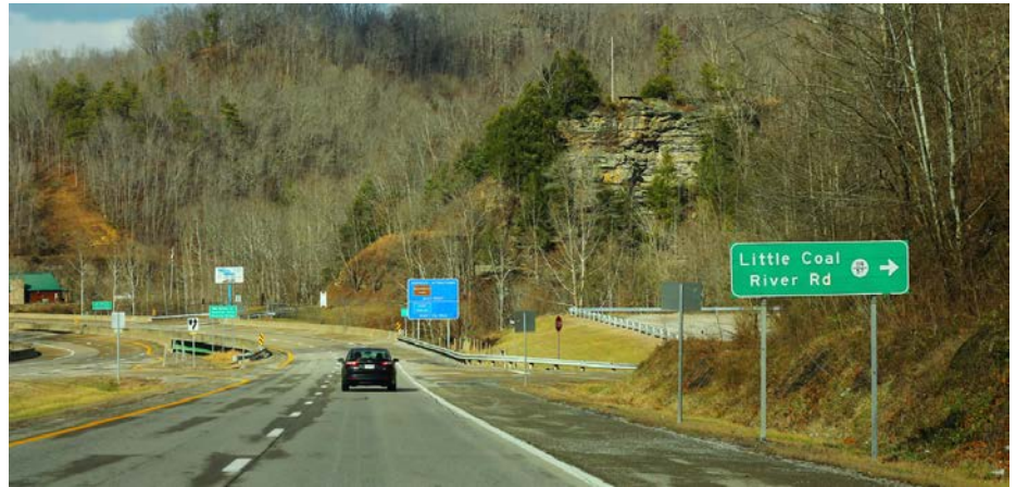
Road users should not be expected to read detailed text on a wayfinding sign while entering a curve. The blue sign should be relocated upstream. © 2017 FormulaNone
