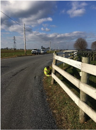
A historic cemetery and edge-of-the road-fixed-objects are some examples of curve complications in PA. (Source: PennDOT)
