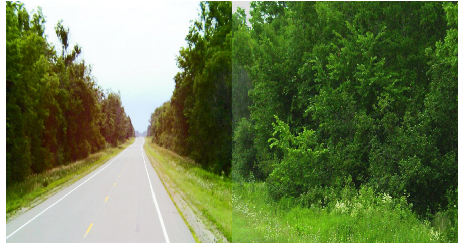
2 - Good Shoulder, No Clear Zone
