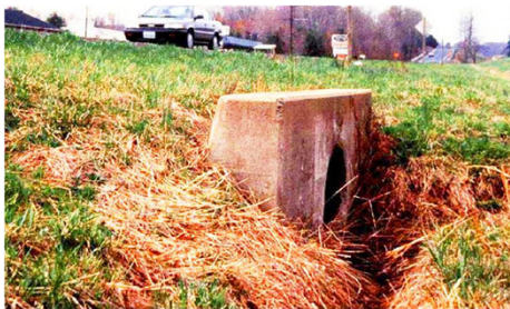
Cross drainage features
