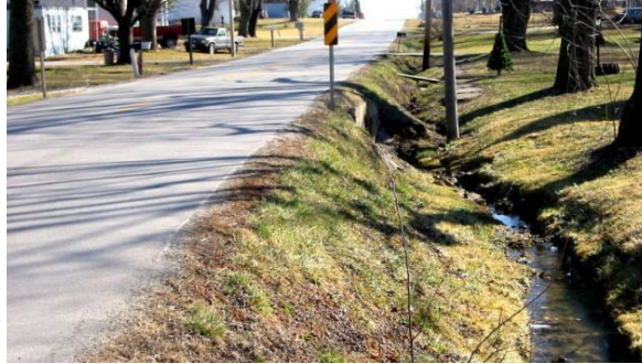
Low Cost Safety Improvements
