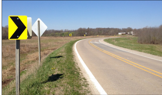
Low Cost Safety Improvements
