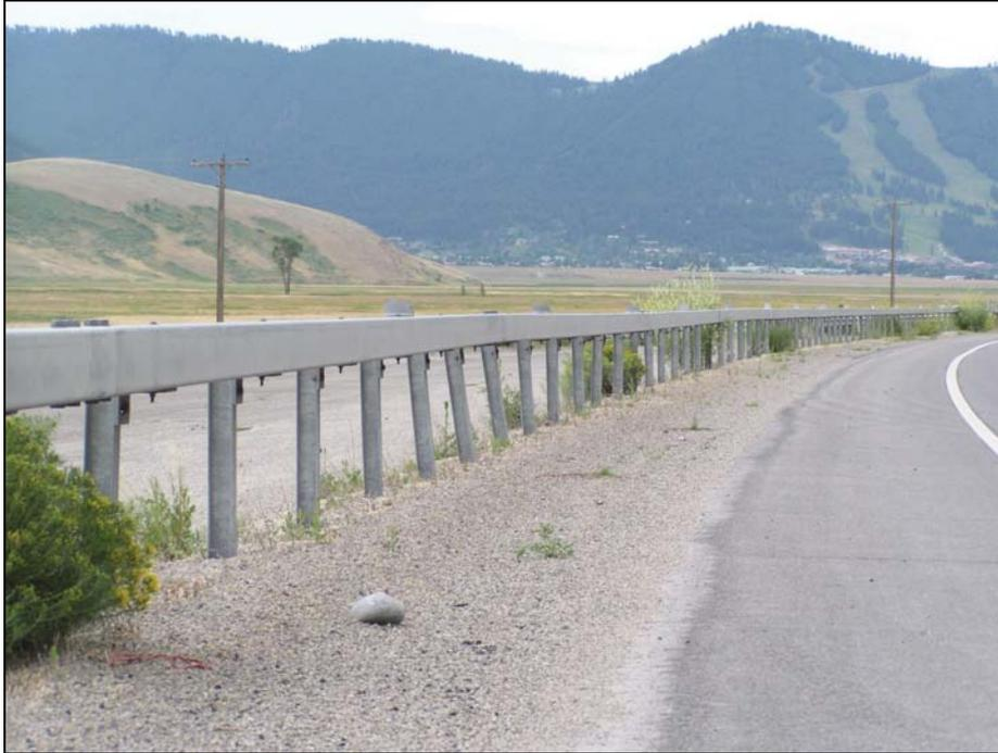
**Table B.6: Strong Post W-Beam, G4****Test Level: 3****Standards Reference:** RDG, M617-10 and M617-11
