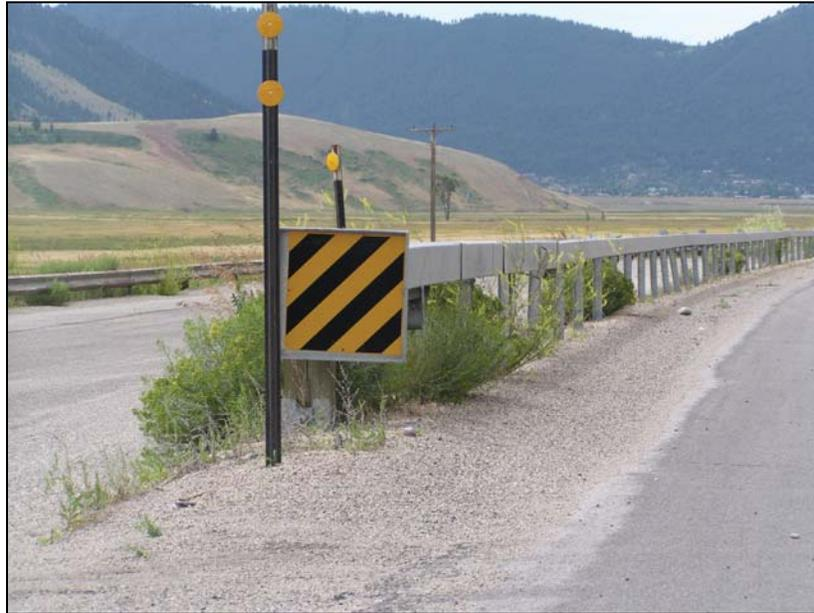
**Figure 3.14: W-Beam with MELT**
