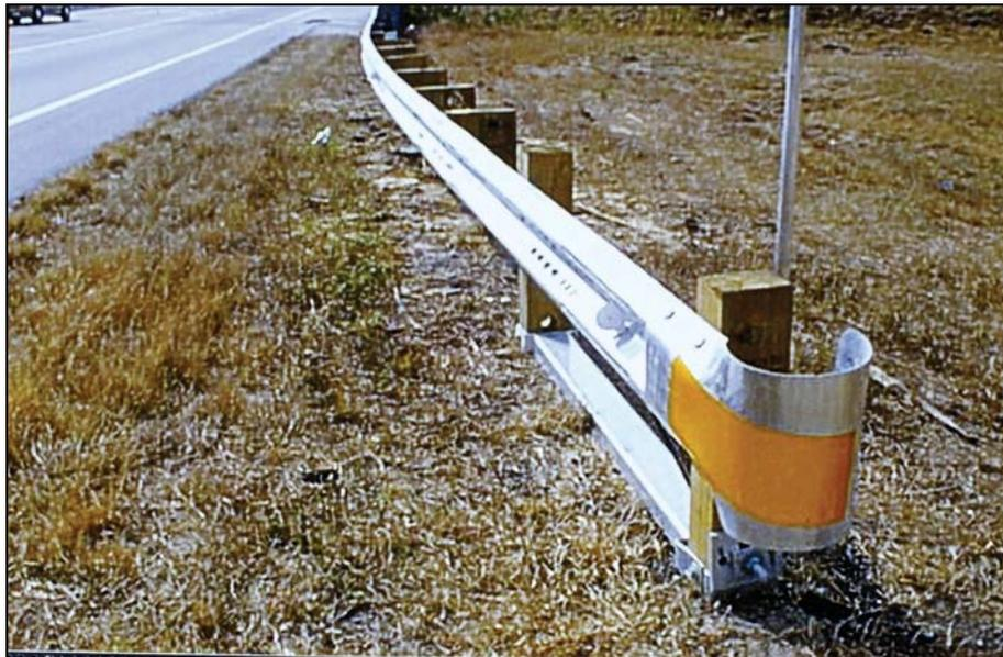
**Figure 3.17: W-Beam Tangent End**
