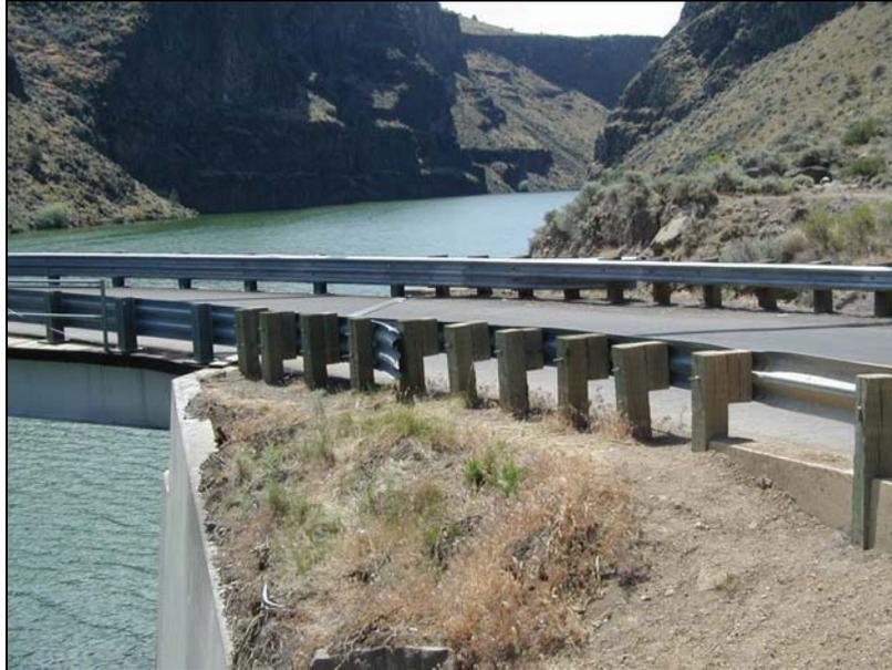
**Figure 3.22: W-Beam to Thrie-Beam Transition**
