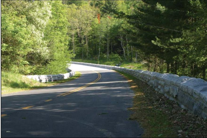
**Table B.14: Random Rubble Cavity Wall, RCW****Test Level: 1****Standards Reference:** Park Service Drawings**Description:** This is a reinforced concrete wall capped with a natural stone and mortar. The wall functions as a rigid vertical faced barrier.
