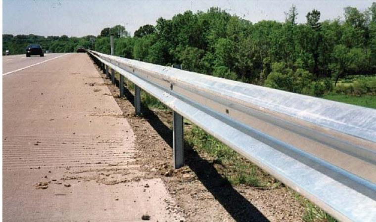
**Table B.5: Box Beam, G3****Test Level: 3****Standards Reference:** AASHTO *Roadside Design Guide*
