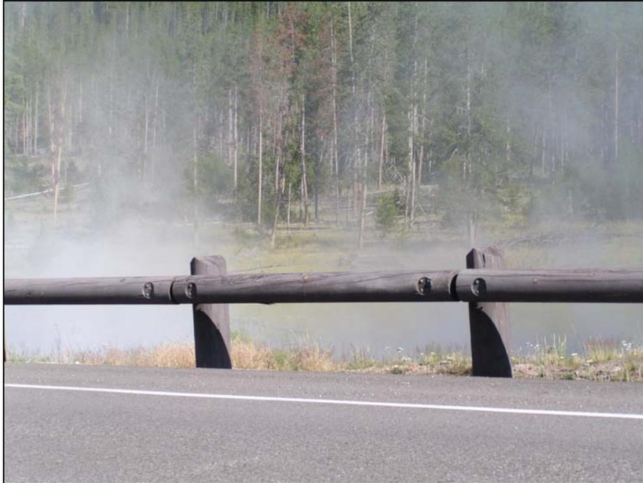
**Table B.11: Steel-Backed Timber Rail, SBT****Test Level: 3****Standards Reference:** M617-60**Description:** This system was developed as an aesthetic alternative. Impact forces are distributed to the posts through the weathering steel plate.
