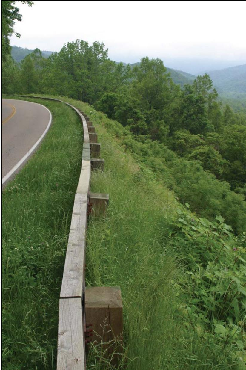
**Table B.12: Precast Concrete Guardwall Type 1, PCG****Test Level: 3****Standards Reference:** M 618-2
