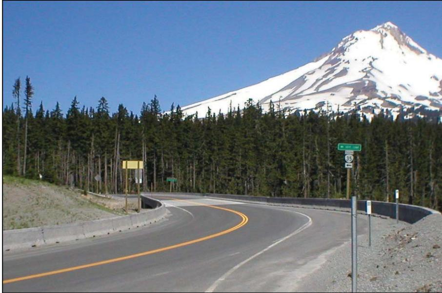
**Table B.10: Steel-Backed Log Rail, SBL****Test Level: 2****Standards Reference:** M617-80 and M617-81**Description:** This system was developed as an aesthetic alternative. Impact forces are distributed to the posts through the steel rail.
