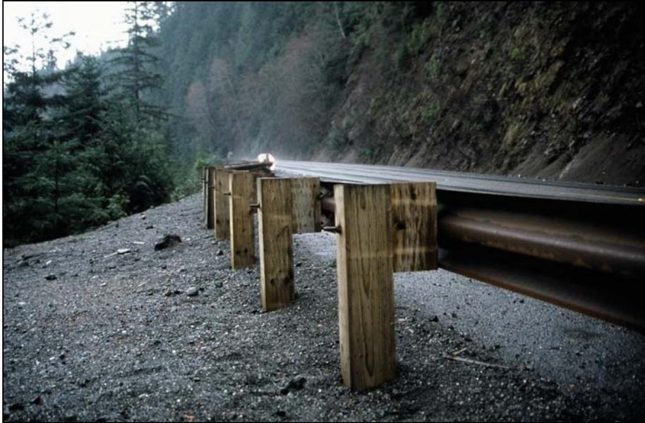
**Table B.7: Thrie-Beam, G9****Test Level: 3****Standards Reference:** AASHTO Roadside Design Guide**Description:** This system is very similar to the strong post w-beam, with the extra depth of the thrie-beam.
