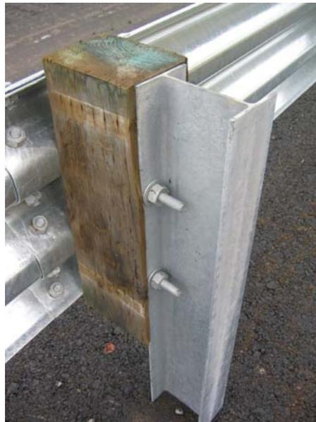
**Table B.8: Modified Thrie-Beam, G9M****Test Level: 4****Standards Reference:** AASHTO *Roadside Design Guide*
