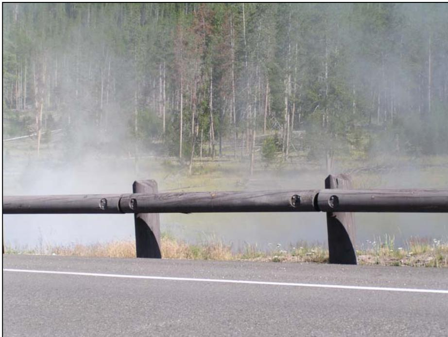
**Figure 3.9: Steel-Backed Timber Rail, SBT**
