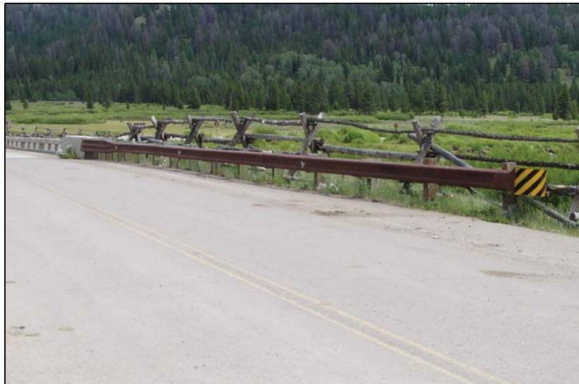
**Figure 3.15: W-Beam Buried in Backslope**
