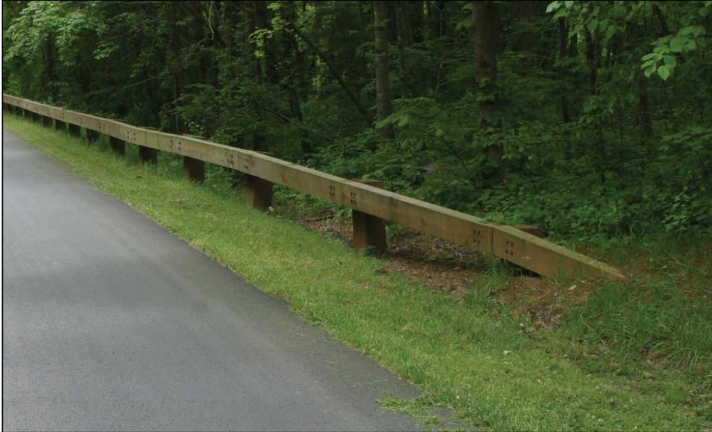
**Figure 3.20: Steel-Backed Timber Buried in Backslope**
