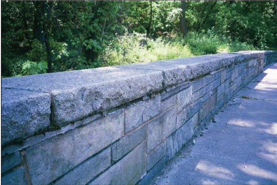
**Table B.13: Stone Masonry Guardwall, SMG****Test Level: 3****Standards Reference:** M620-1
