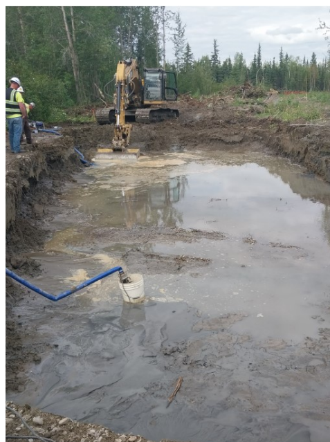
Left: Ground water sub excavation on Lathrop St.
