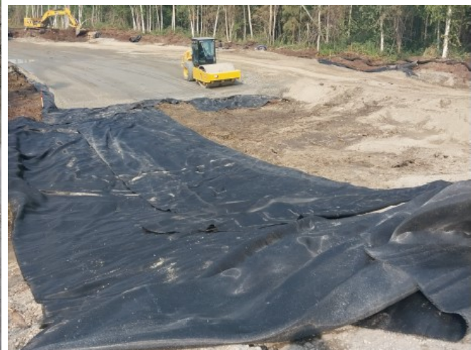
Below: Placing Select Borrow on Northlake Lane.
