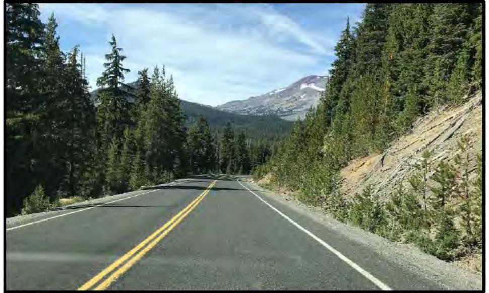
Typical roadway view of CLH – narrow shoulders, areas of limited horizontal sight distance along horizontal curves
