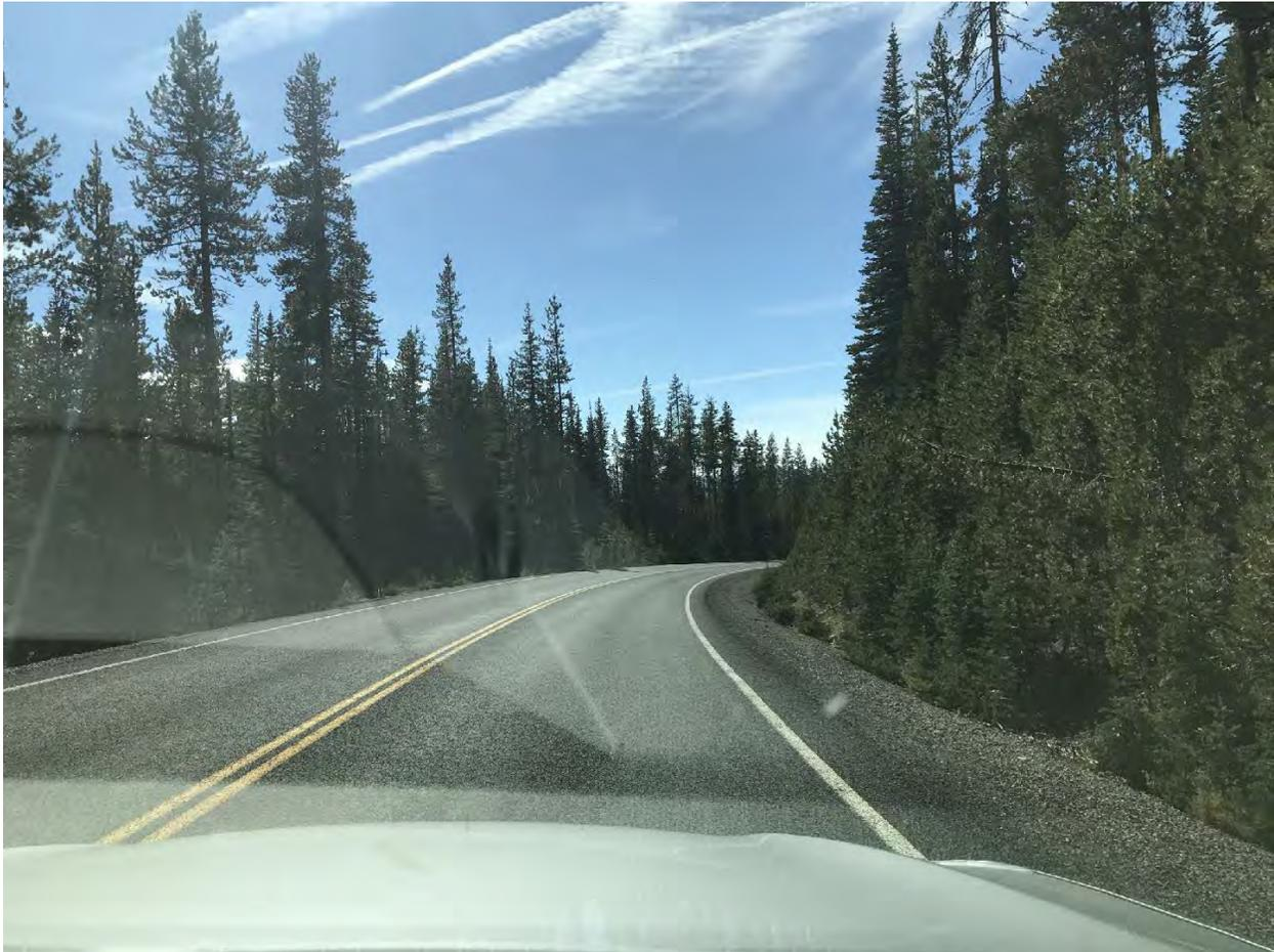
*Figure 11 - Limited Horizontal Sight Distance*
