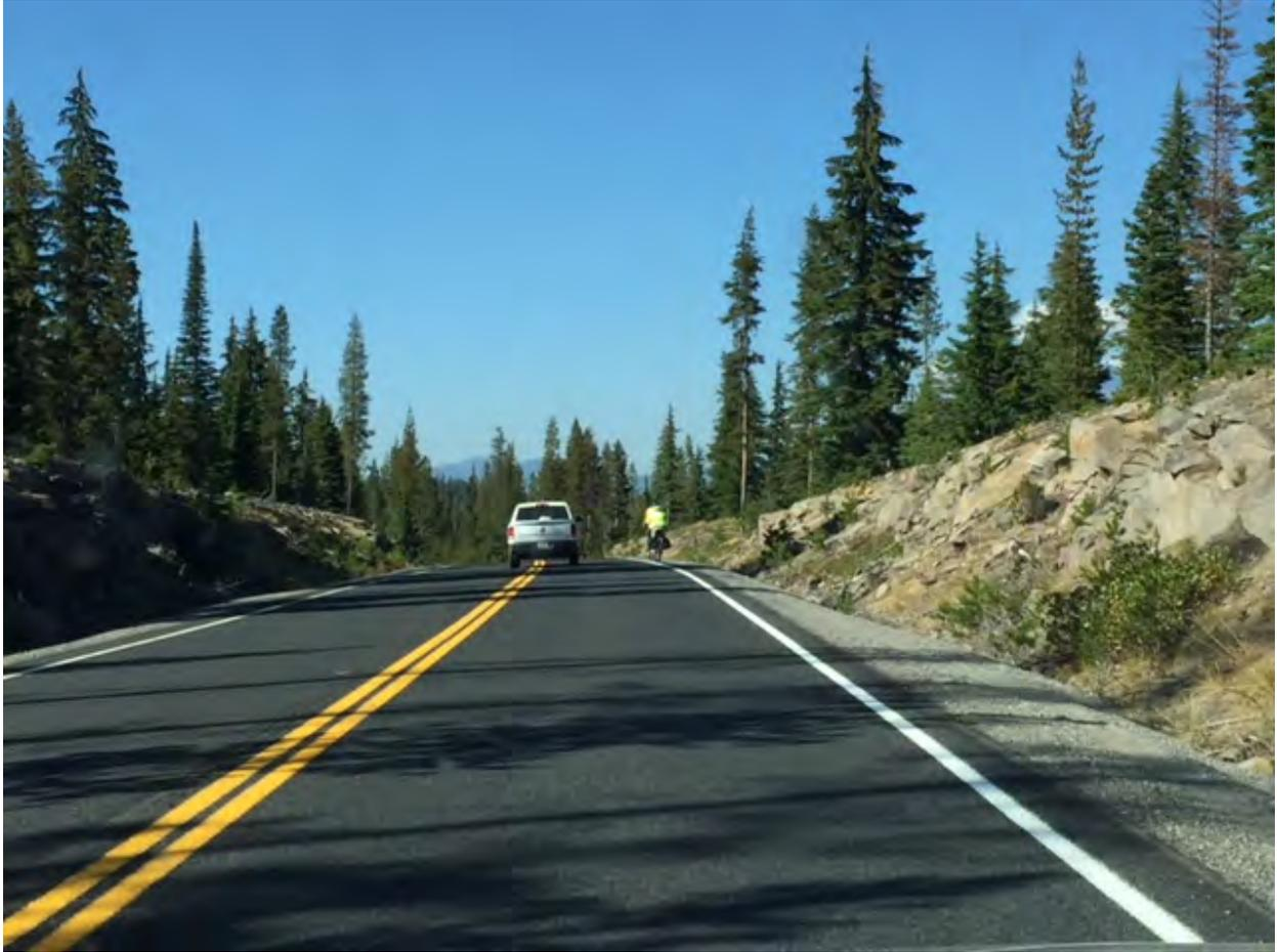
*Figure 8 - Motorist Passing Cyclists in Area of Limited Vertical Sight Distance*
