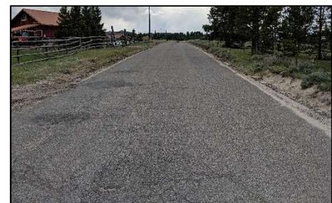
*There are several locations where the pavement experiences failures including cracking, potholing, flushing, rutting, distortion, edge erosion, and failing patches.*
