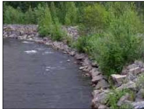
*Riprap would be placed along streambanks to control the flow of Blacktail Creek, stabilize the banks, and prevent further erosion on Roosevelt Drive.*
