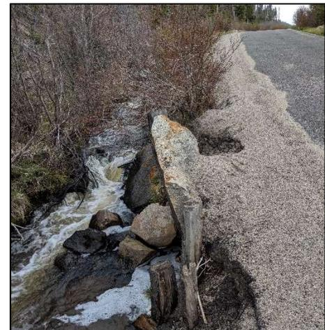
*Culverts help control drainage to reduce erosion. About 45 percent of culverts in the study area are in poor condition.*
