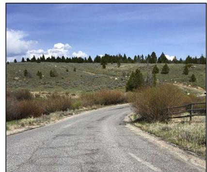
*Between MP 2.2 and 2.4 there is an s-curve with tight combination horizontal/vertical curves. The steep cut slope, vegetation, and parking along the road limits sight distance at this location.*
