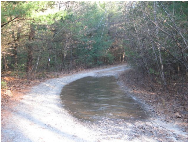
Example of ponding on Harry's Way
