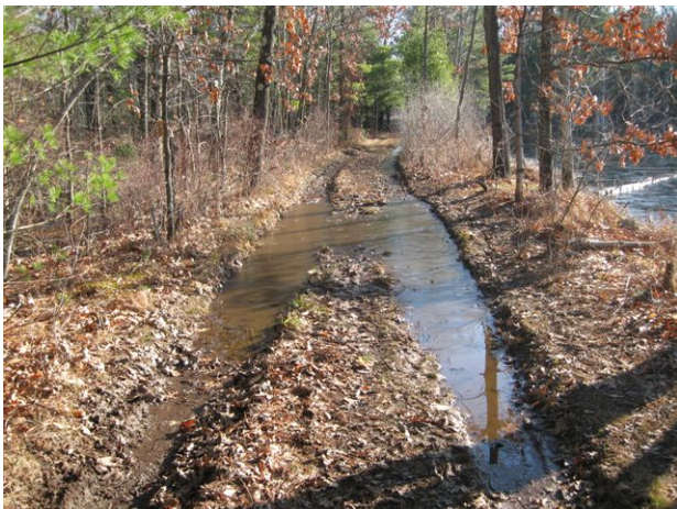
Ponding in tire ruts along Otter Alley.
