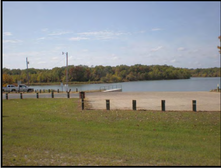
Figure 3.12: Port of Crossett Boat Ramp
