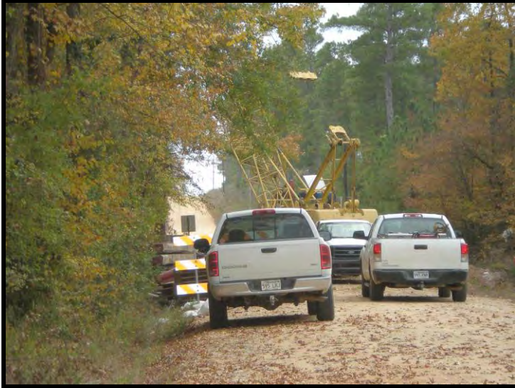
Figure 3.7: Bradley County Road 53
