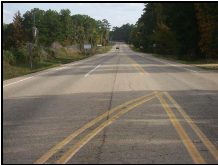
Figure 3.14: Left-Turn lane into Visitors Center
