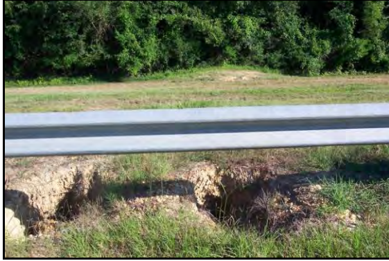
Figure 5.8: Voids along Embankment (Typical)
