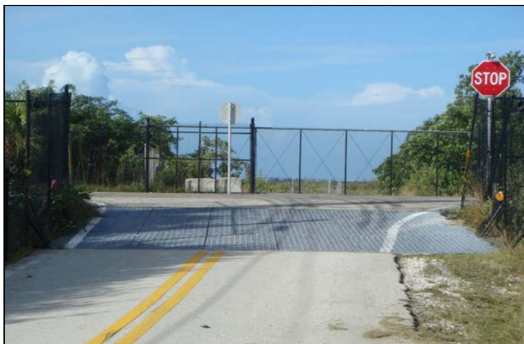
Figure 4.3: Example of Key Deer Grates in Fenced Areas
