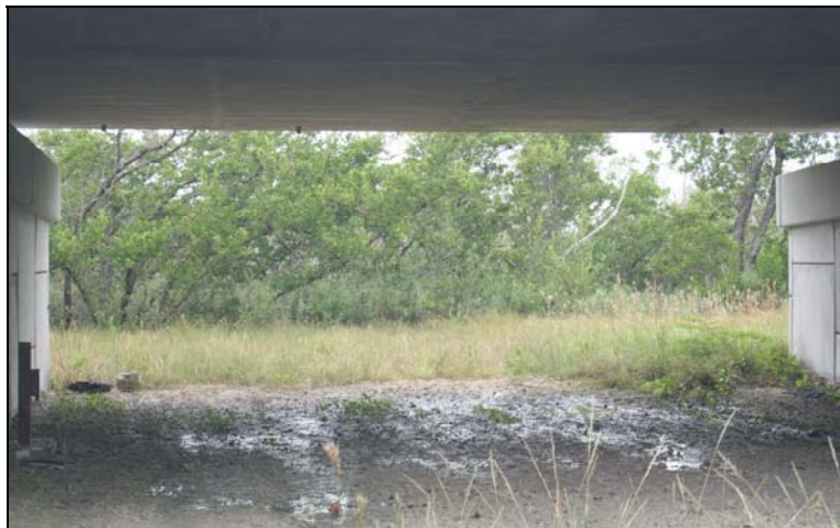
Figure 4.2: Example of a Key Deer Underpass
