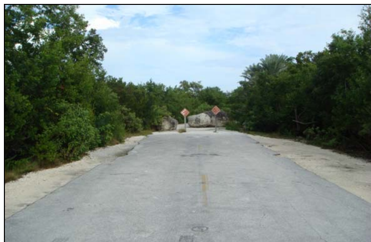
Figure 4.8: Gravel Shoulder at Watson Boulevard Terminus on No Name Key
