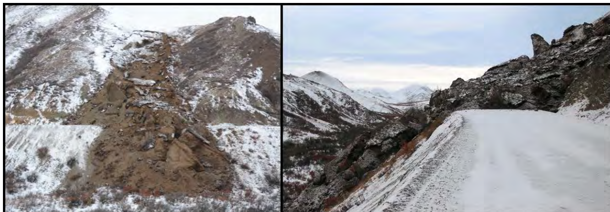
Figure 2: Igloo Creek Landslide on Denali Park Road (Source: WFL).
