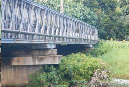
Pier at Wainiha Bridge 3
