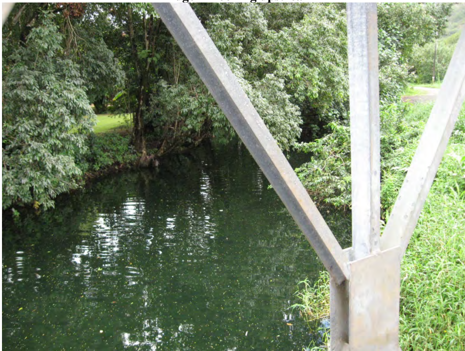
Bridge #2 looking upstream
