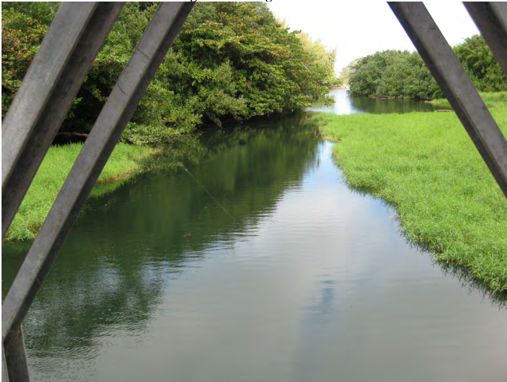
Bridge #3 Looking downstream
