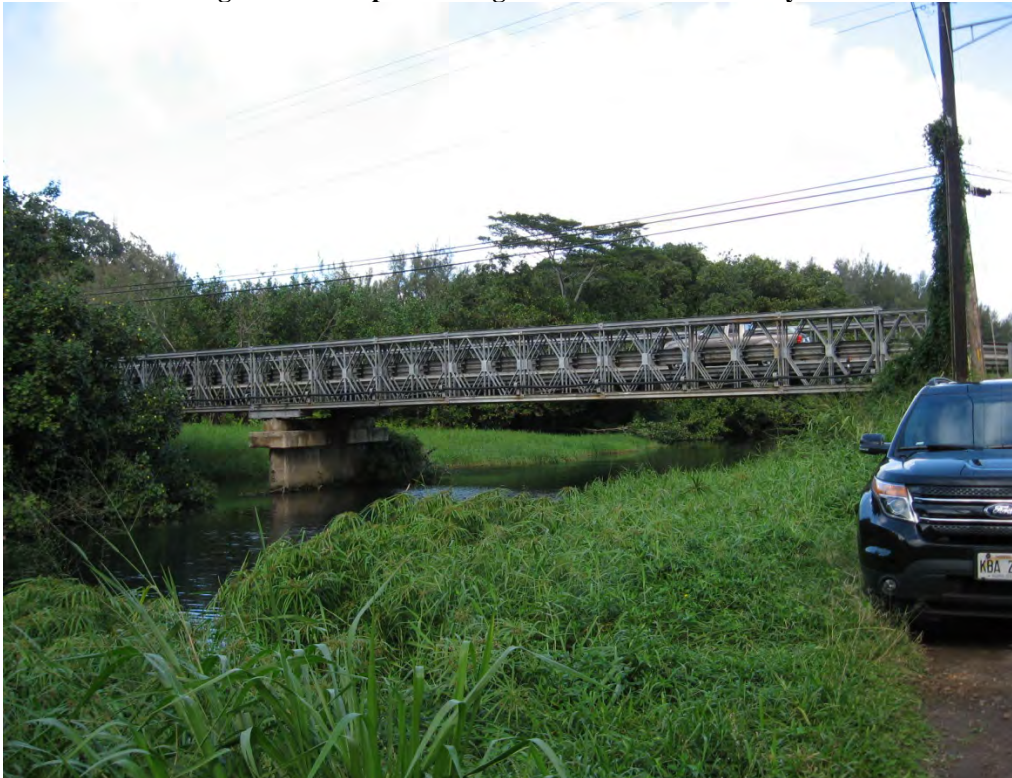
Bridge #3 Lihue Span looking downstream from county road
