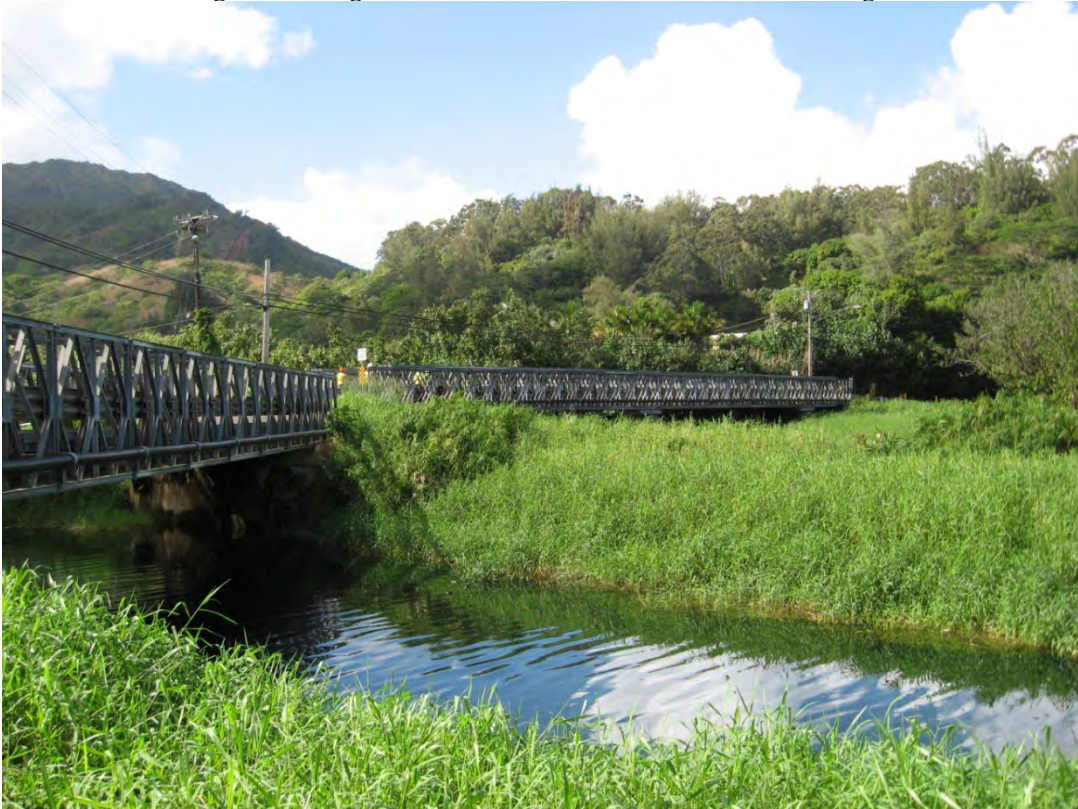
Bridge #3 looking at downstream side from Lihue end of Bridge #2
