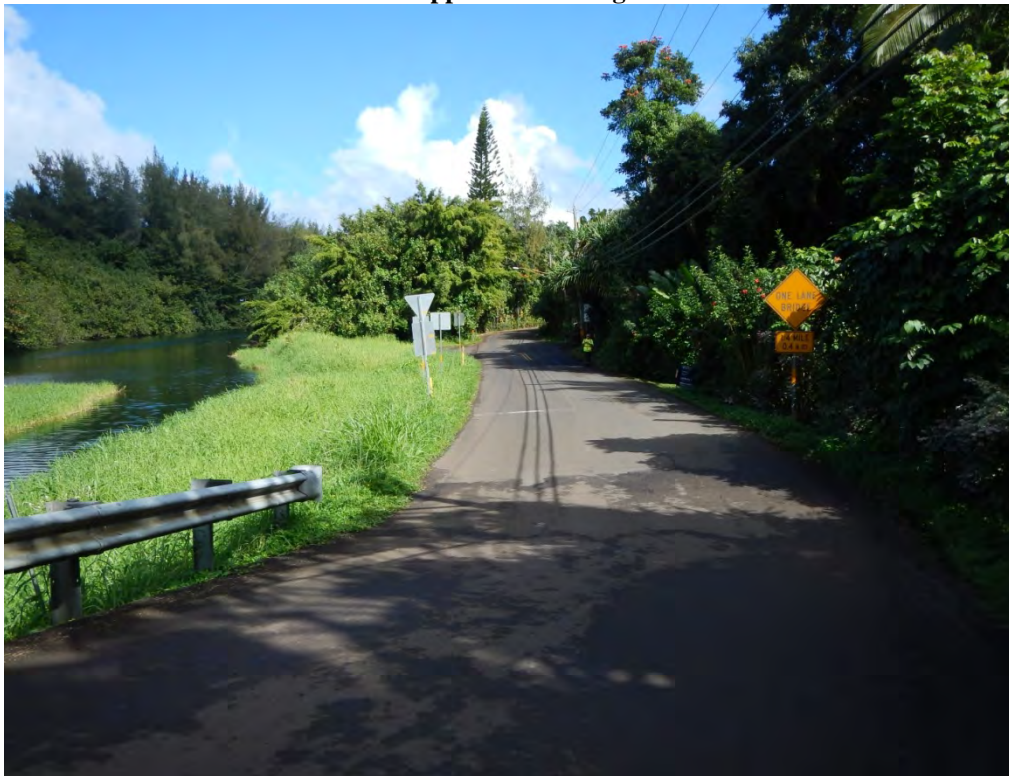
East approach to Bridge 2
