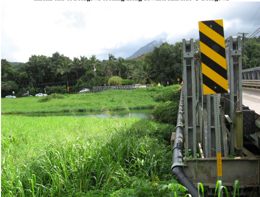
Haena end of Bridge #3 looking along downstream side @ Bridge #2
