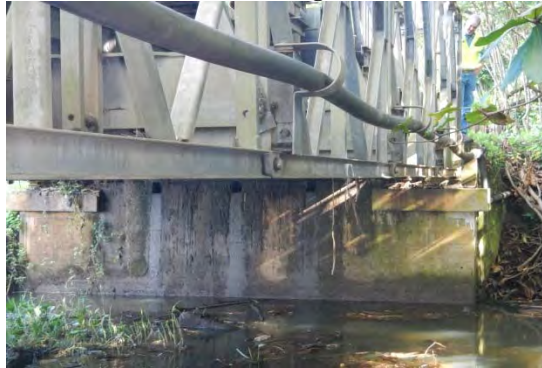
Abutment at Wainiha Bridge 1
