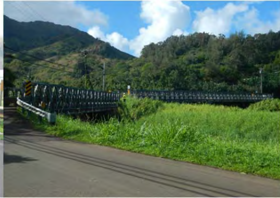
Wainiha Bridge 2 and Bridge 3
