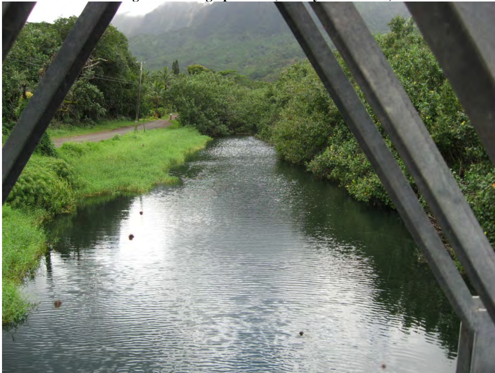
Bridge #3 Looking upstream (County road on left)
