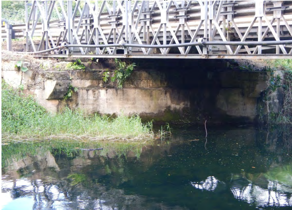
Upstream of Bridge 2 looking at east abutment
