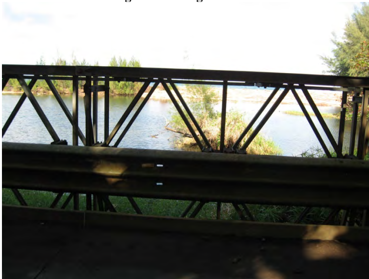
Bridge #1 Looking downstream
