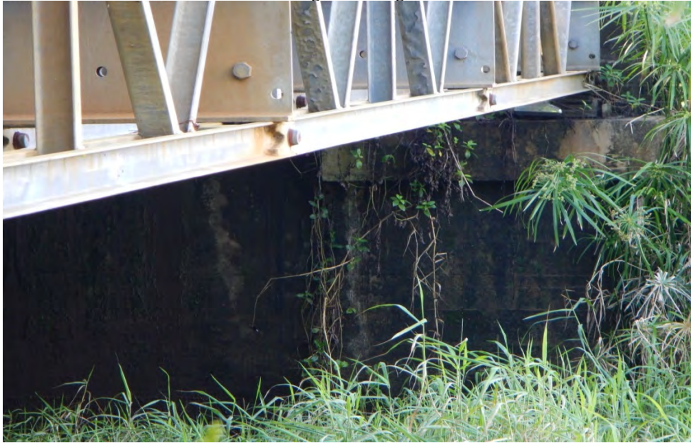
Downstream of Bridge 1 looking at west abutment
