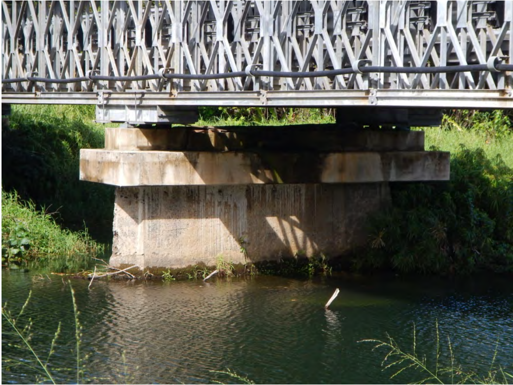
Upstream of Bridge 3 looking at east pier
