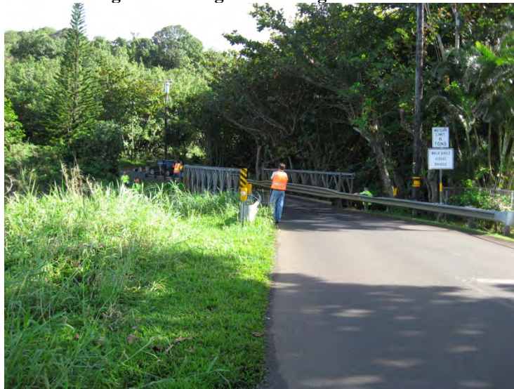
Bridge #1 Looking across bridge toward Lihue
