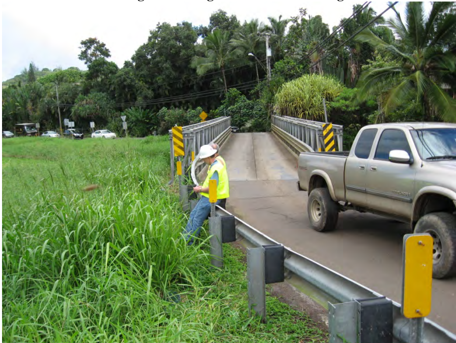
Bridge #2 looking at Haena end of bridge
