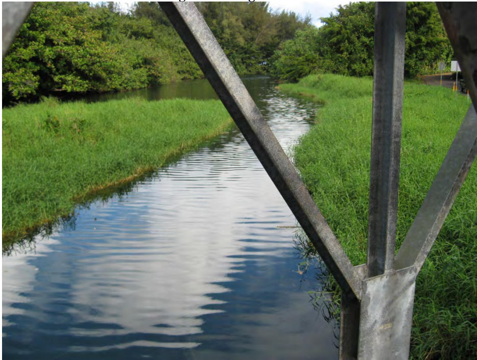
Bridge #2 looking downstream
