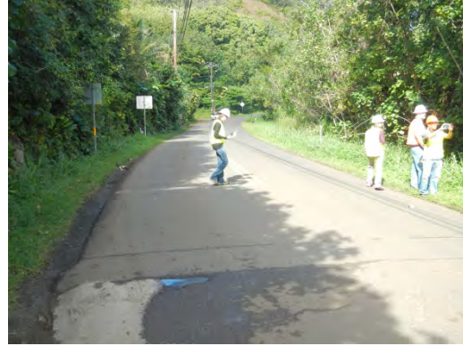
Pavement Conditions near Bridge 3
