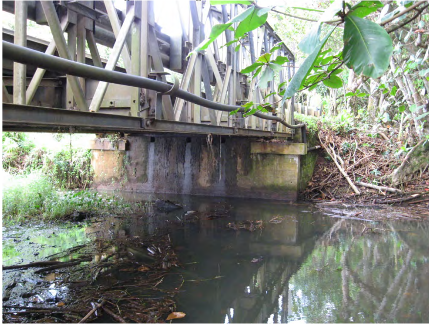
Bridge #1 Looking at Lihue abutment wall
