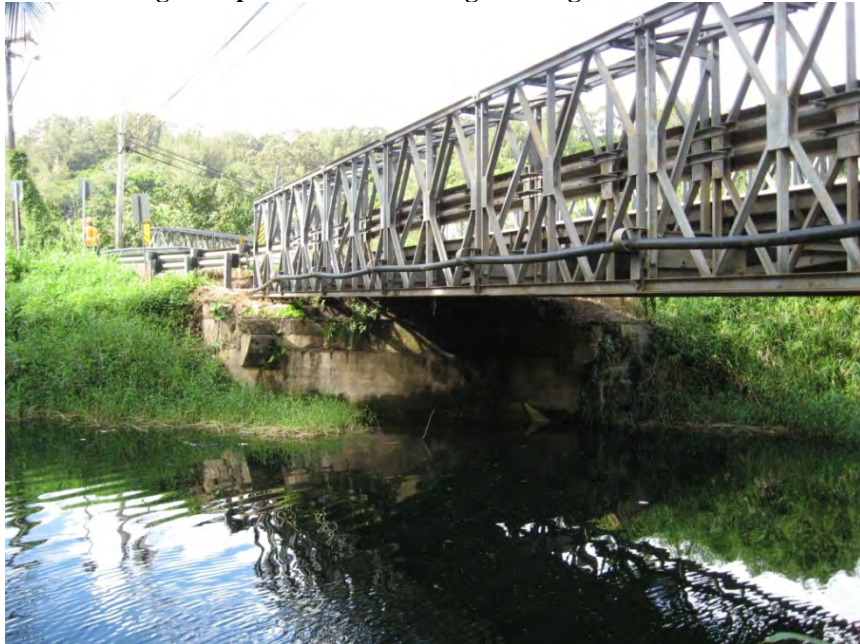
Bridge #2 upstream side of bridge looking from Lihue end
