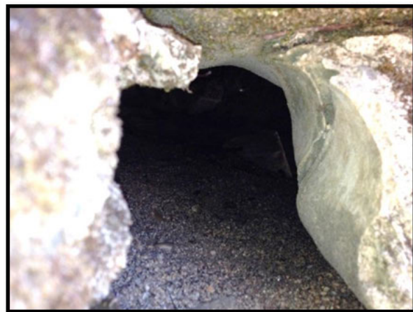
Photos #12, 13 – Void in Cement Bag Wall (Abutment 2)
