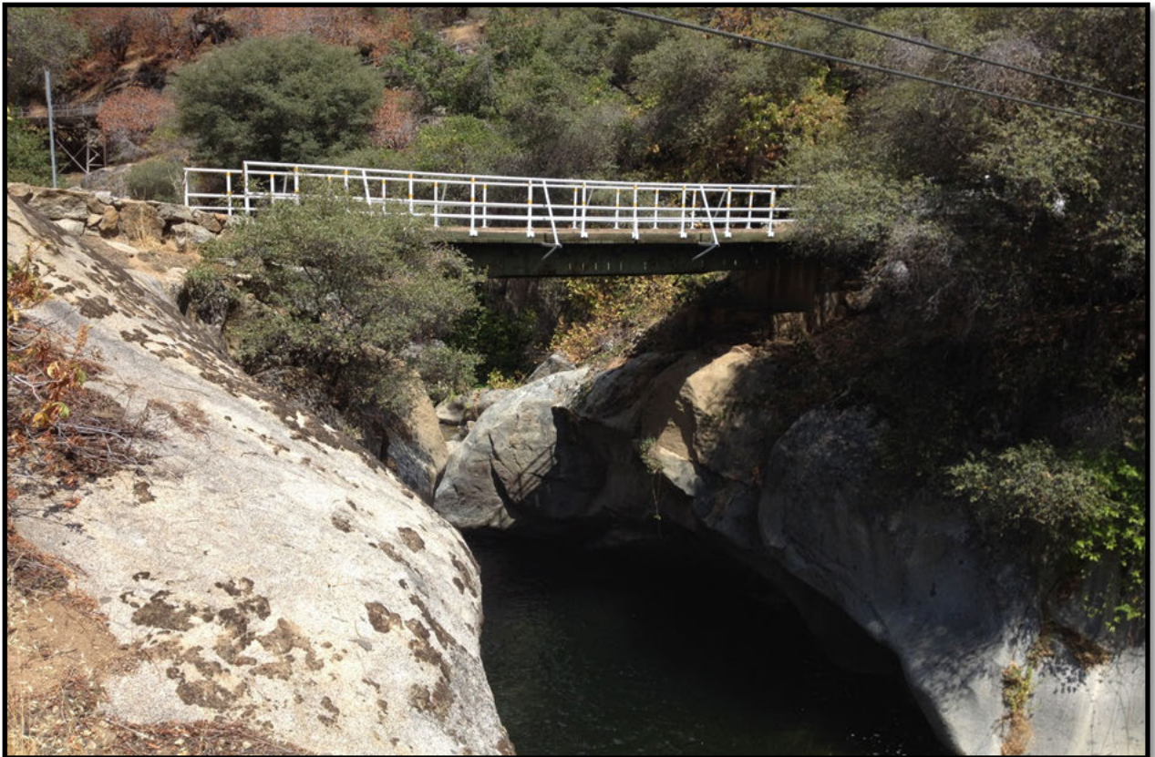
Photo #4 – Bridge profile (looking upstream)
