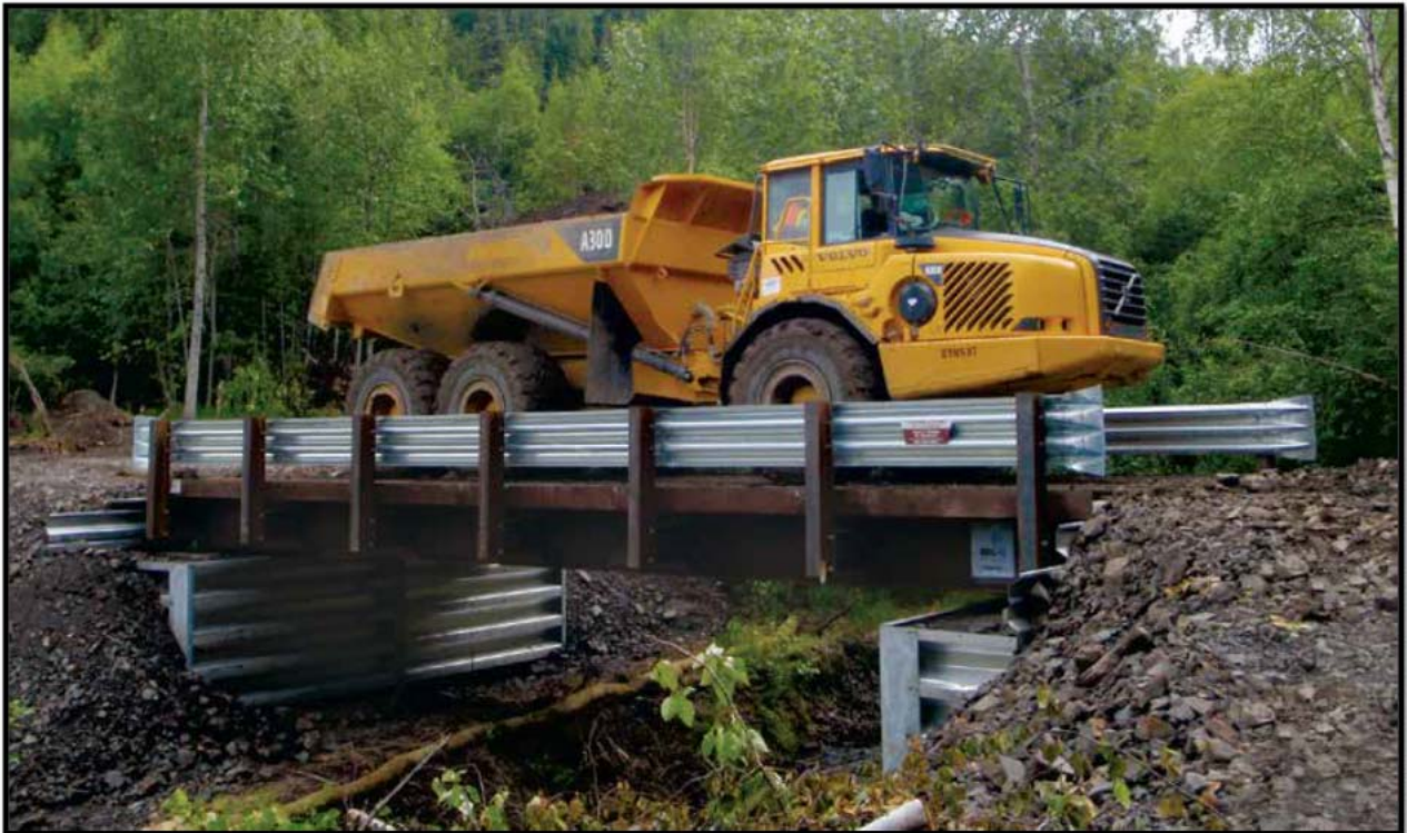
Photo #10 – Bridge Railing Flared End Treatment
