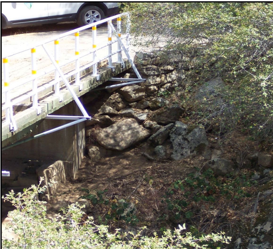
Photo #8 – Abutment 2 downstream wingwall
