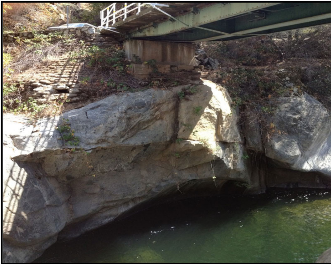
Photo #6 – Abutment 2 (South)
