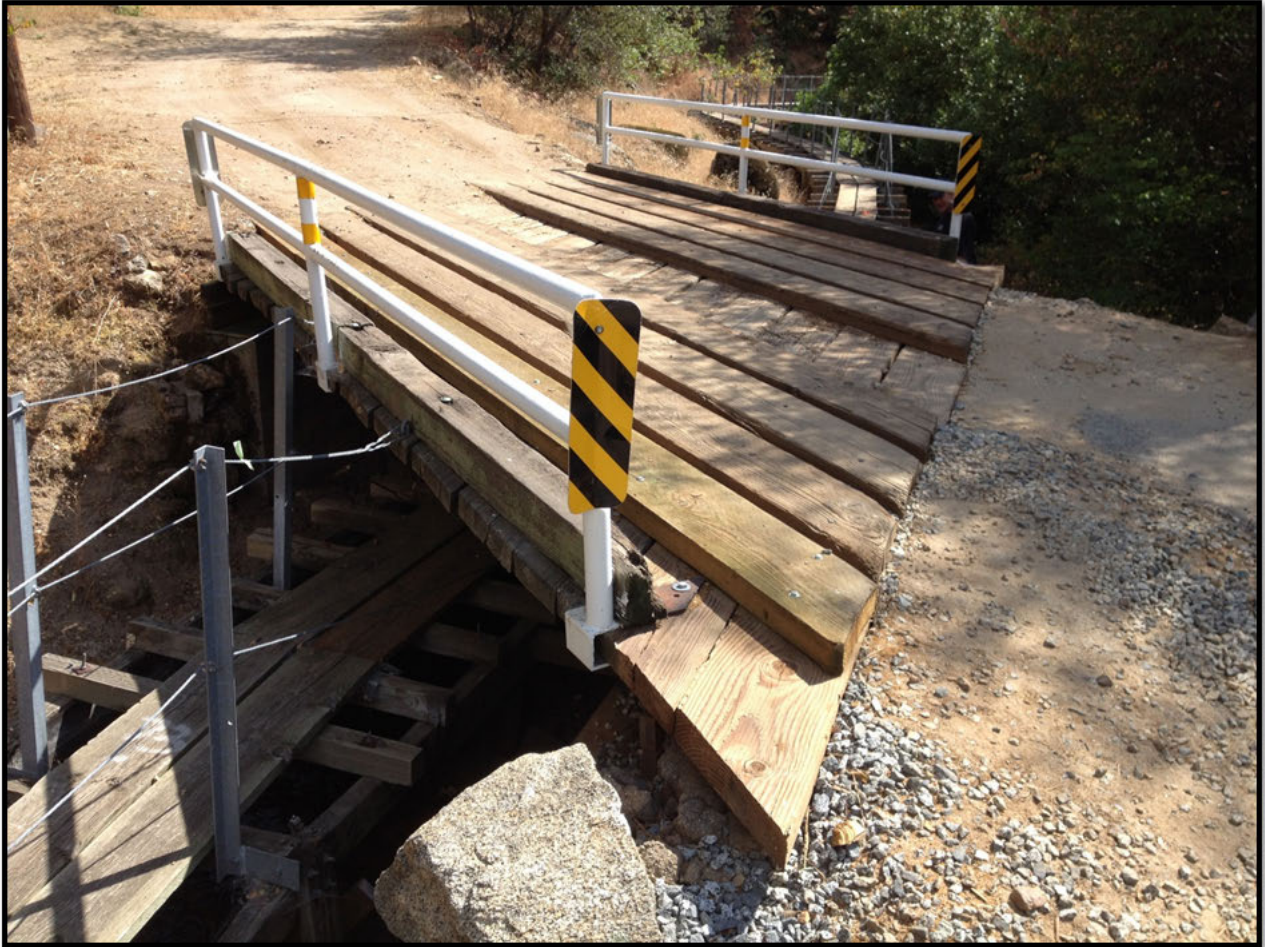
Photo #9 – Kaweah Flume Bridge
