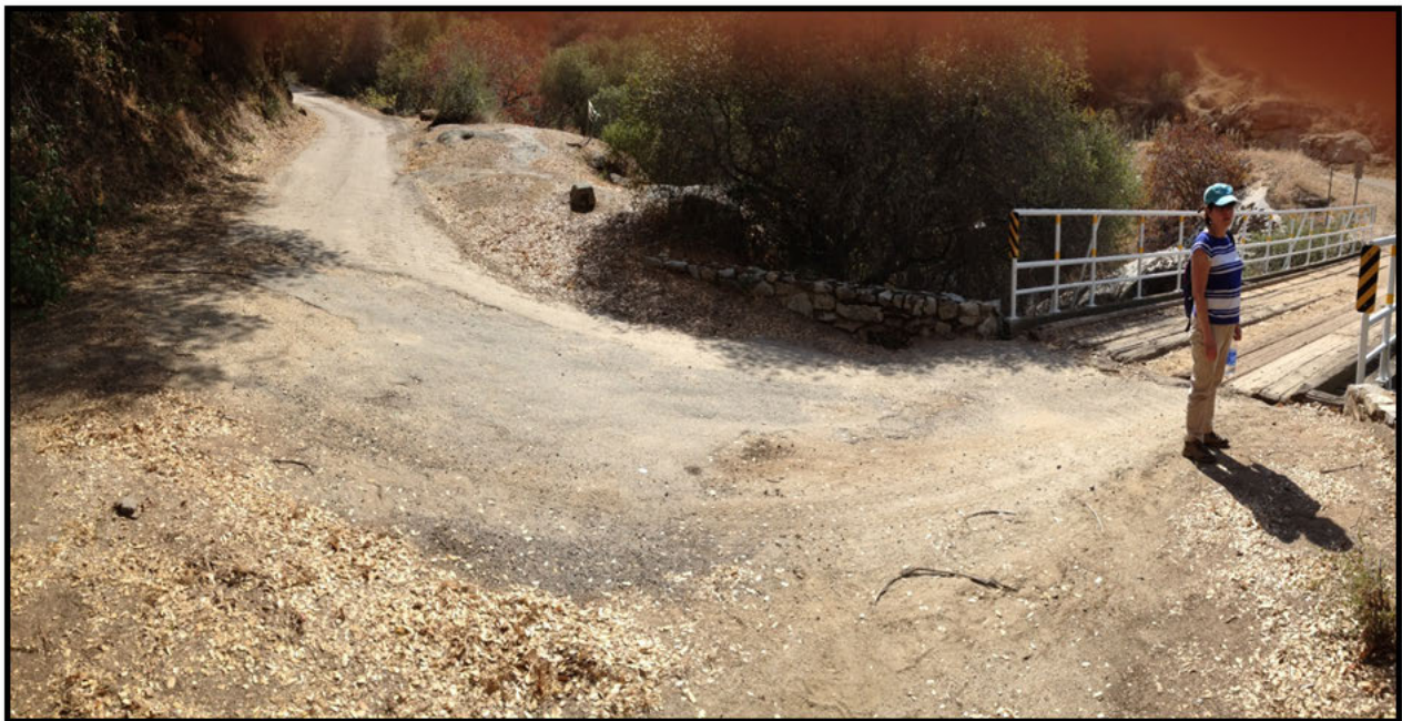
Photo #2 – South approach
