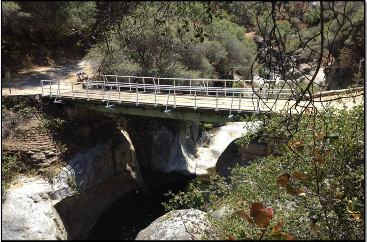
Photo #3 – Bridge profile (looking downstream)
