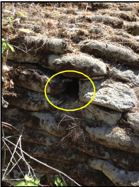
Photos #12, 13 – Void in Cement Bag Wall (Abutment 2)
