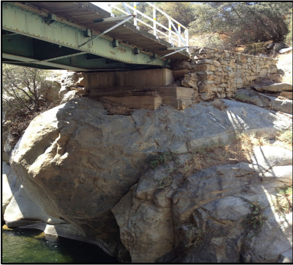
Photo #5 – Abutment 1 (North)
