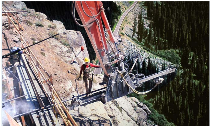
To stabilize the fractured rock of the cliff, the contract requires four rock anchors to be installed. Here, the contractor drills a horizontal hole for one of the anchors. The drill is mounted on the boom of an excavator, which stands on the roadway above. Below is a lower level of Highway 410.
