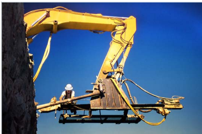
The drill on the boom of an excavator. When the hole is complete a 25-foot-long anchor will be installed; grout will be injected around the anchor to hold it in place.
