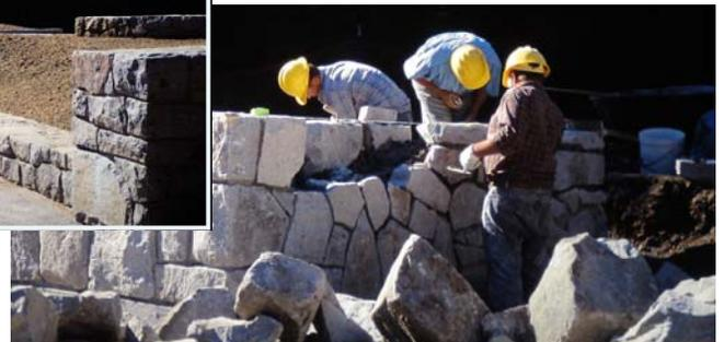
Stonemasons fit the shaped stones together and apply mortar. Inset: Completed stone wall at Fife's Peak Overlook. Photos courtesy Gary Hunter
