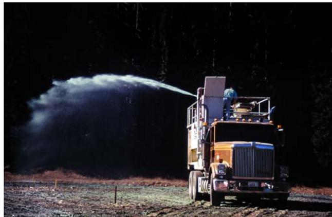
A hydroseed truck shoots a mixture of water, grass seed, fertilizer, and mulch over the topsoil on the reclaimed borrow pit. Photo courtesy Gary Hunter
