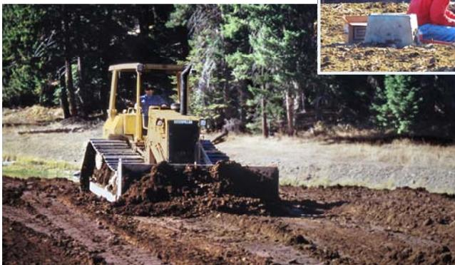
With the irrigation system working properly, the subcontractor places topsoil over the recontoured borrow pit.
