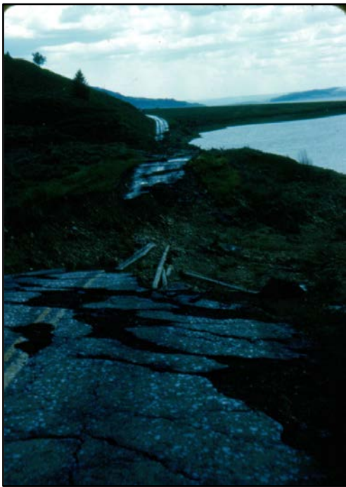
Mat and roadbed slide caused by earthquake. Photo by Rexford G. Reilly.
