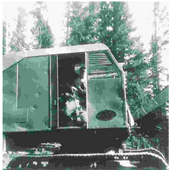
Pile driver (and operator “Red”) at Yellowstone National park, 1961. Photo courtesy Larry Brown.
