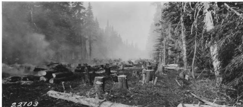
The initial clearing for a road through timberland: This section shows the final burning during a contract on Santiam Pass, Oregon, June 28, 1932. From the final construction report, Santiam Pass, Suttle Lake, No. 23-E1, 23-G and 23-D2, F. WFLHD Archives.
